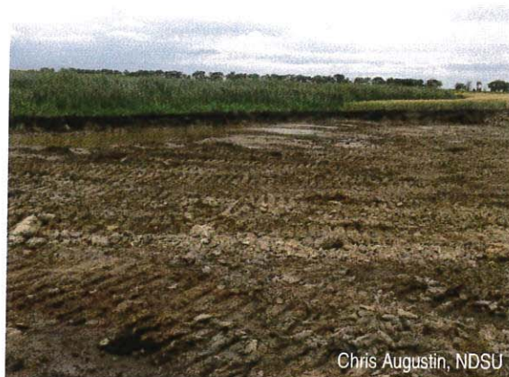
Figure 6. The topsoil was removed from this spill site as part of ex situ remediation.
