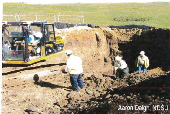
Figure 6. The topsoil was removed from this spill site as part of ex situ remediation.
