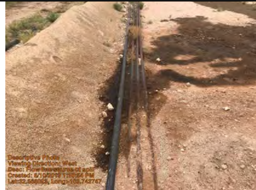
Flow line source of spill
