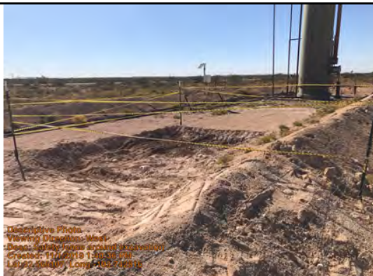
Safety fence around excavation
