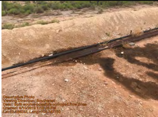
Spill source-possible corroded flow lines
