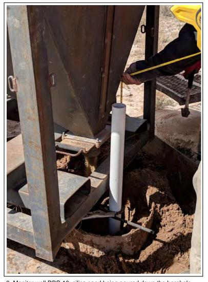
6. Monitor well DBS-10: silica sand being poured down the borehole, extending from bottom of borehole to approximately 5 feet above the top of well screen. Bentonite chips were then placed on top of the silica sand filter pack, extending to depth of 15 feet bgs. Cement grout was then used to fill the remainder of the annulus.
