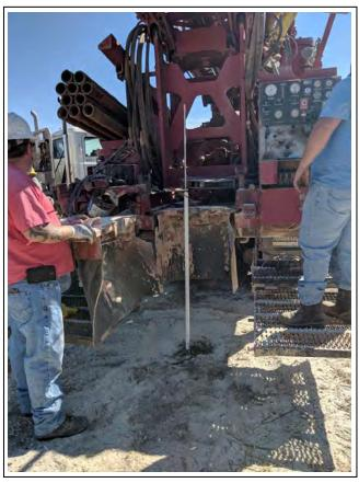
Installation of survey monument SMP-3. The monument was centered and suspended within the borehole, and the anchor plate and sleeve were carefully placed before installing cement grout to anchor the monument in sandstone.
