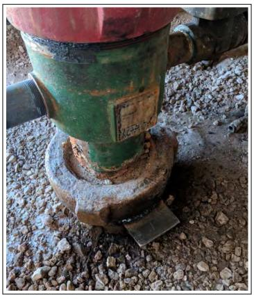
4. Survey monument SMP-5, consisting of a stainless steel plate welded directly onto the brine well casing.
