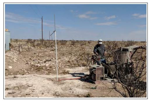
3. Installation of survey monument SMP-1: anchor plate being grouted. Sand was then placed on top of the grout to fill the annular space. Then the sleeve was cut and grouted at the land surface.
