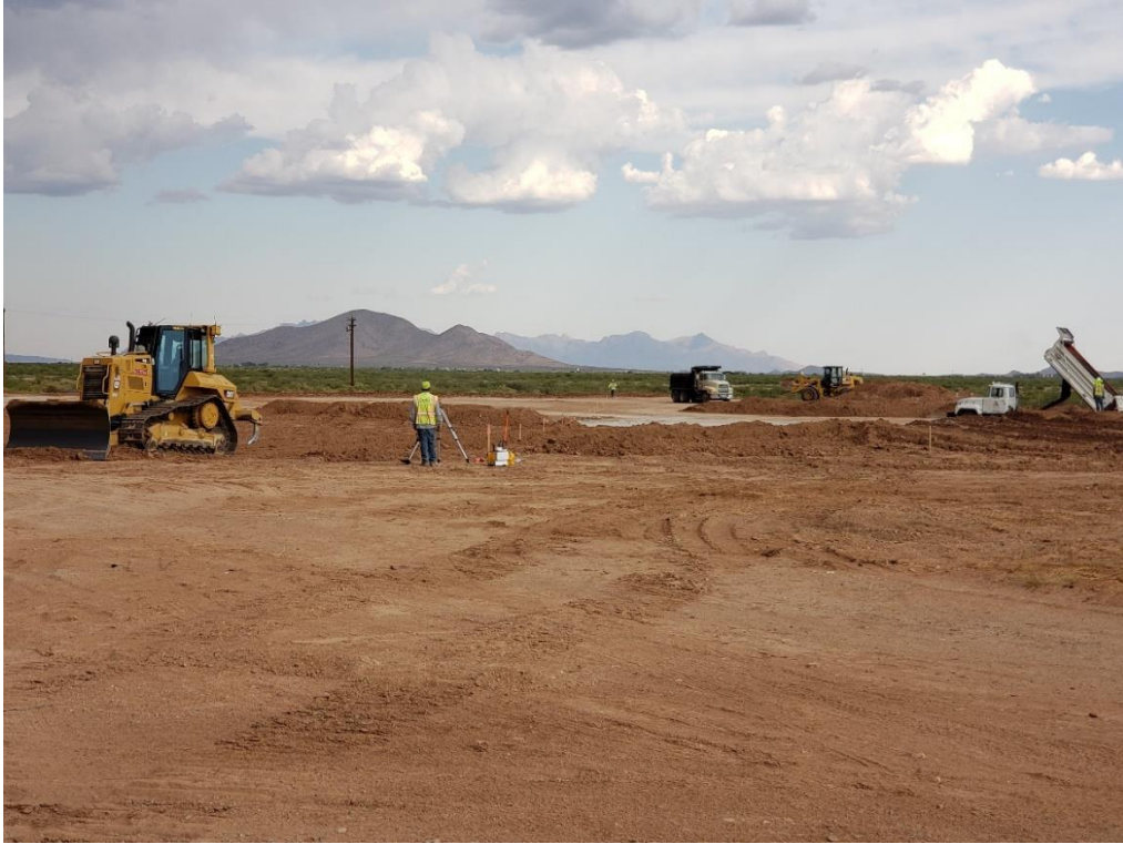
Photo 11: Staking survey to determine grade
