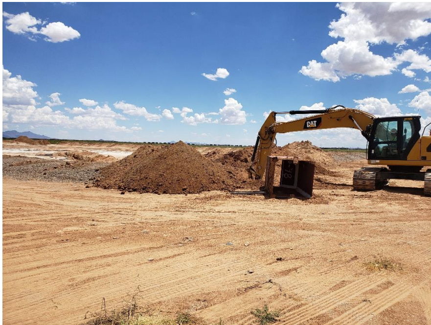
Photo 6: Excavation of drain line valve box
