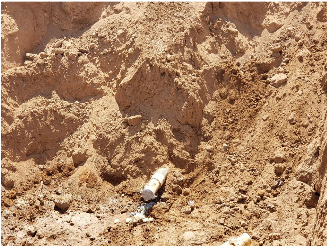
Photo 8: Drain line cut and plugged with concrete
