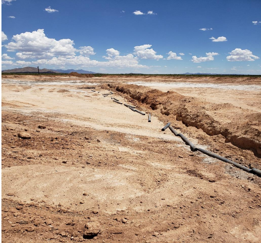
Photo 5: Excavation of 2-inch drain line beneath pond liner
