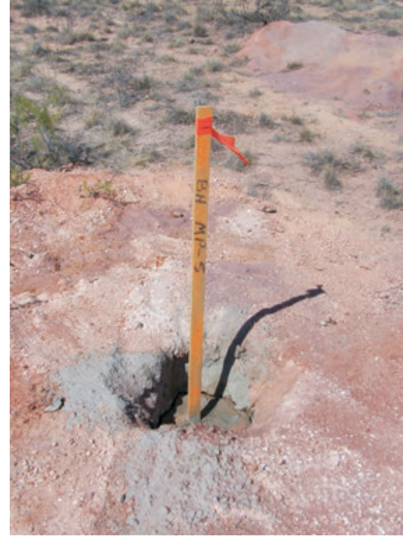
Photograph 22. Boring MP-5 plugged using cement-bentonite grout slurry (also typical of other borings).
