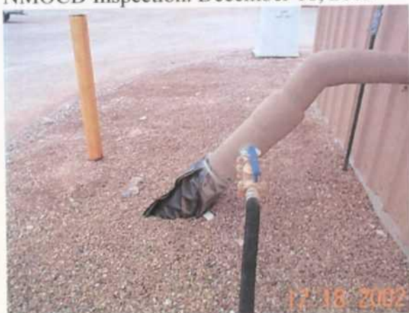
Photo 12: Transfer pipe from truck unloading area to tank area is below grade. Below grade portion of the pipe is wrapped and sealed with a 60 mil liner.
