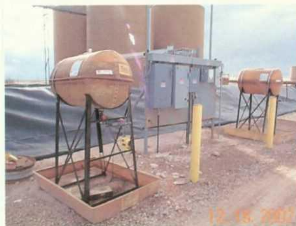
Photo 3: Saddle tanks labeled as to contents and warnings. Tanks have secondary containment.
