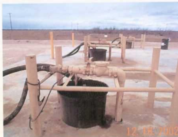
Photo 14: Above-ground poly sumps on concrete pad.
