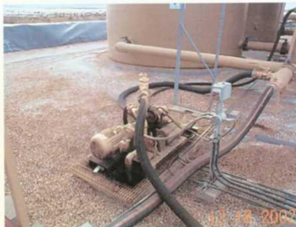
Photo 4: pump with secondary containment inside lined bermed area. Tanks on gravel rings.
