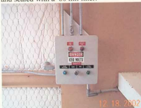
Photo 13: Key only unloading system. If the tank levels set at 5 feet go off the unloading system will not allow trucks to unload.
