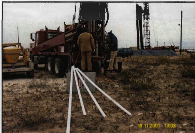
Photo 2. View of PVC used for MW-1. Date: 19 November 2001.
