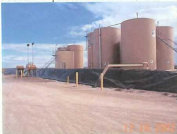
Photo 1: 60 mil lined tank storage area. Berms are 5 feet high.
