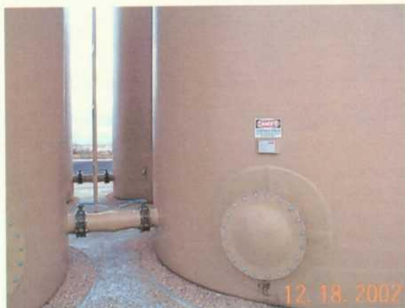
Photo7: Confined space entry warnings were on all tanks. All tanks were on gravel rings.
