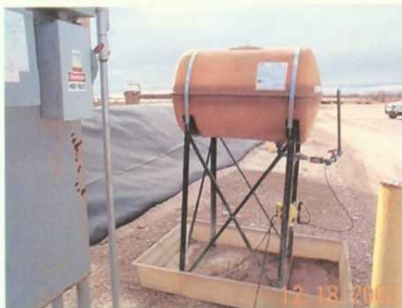
Photo 2: Saddle tank labeled and contained.
