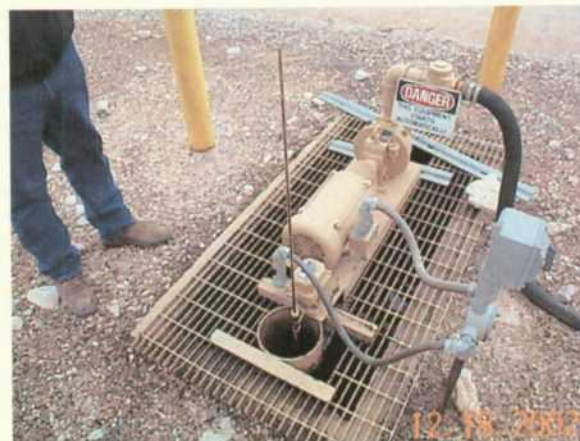
Photo 11: Single walled sump for truck runoff or spills. Automatic sump-pump removes liquids.
