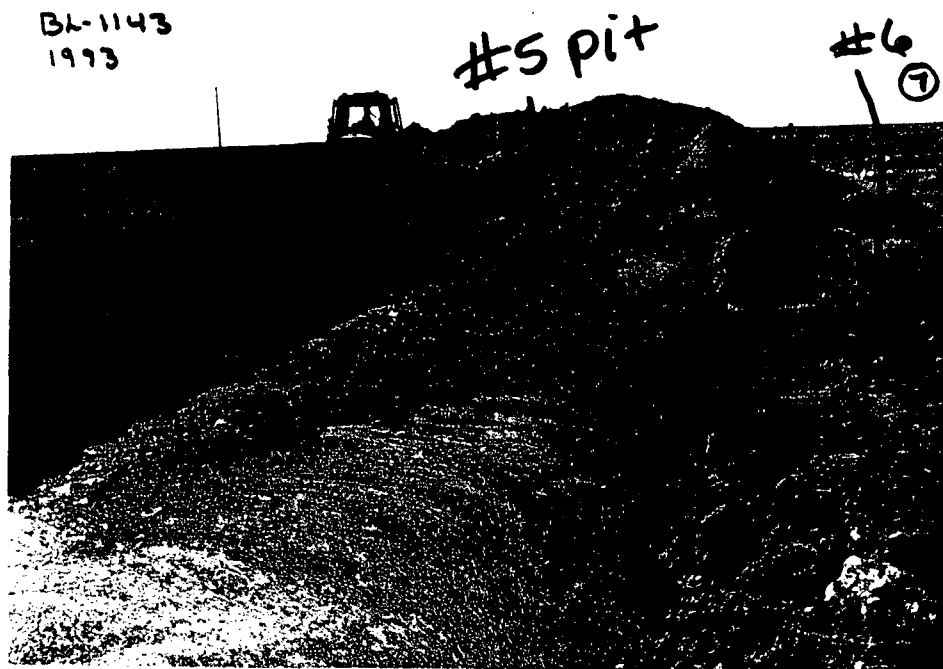
Picture #7 #5 PIT, 15' DEEP, 100% WASTE MATERIAL, #6 PIT PRIOR TO REMOVAL OF DIRT
