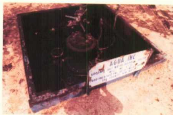
Photo 6 Agua Inc. Injection well and celler
