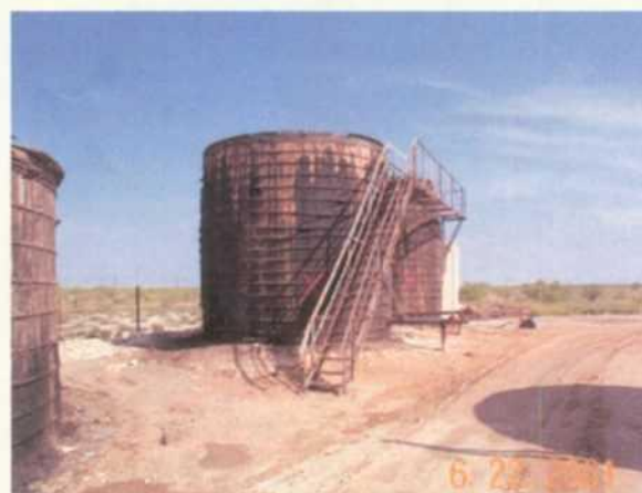
Tank 111 in foreground with red x ( 30.8 \pm 0.86 pCi/g March 2001). Tank 112 behind tank 111 with red x ( 48.8 \pm 1.24 pCi/g March 2001) ( 47.28 \pm 2.50 pCi/g October 2000).
