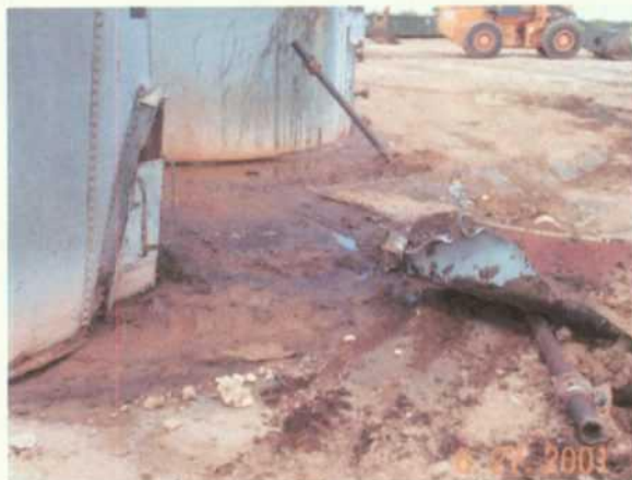
Tank removal. Tanks have leaked, looking east.
