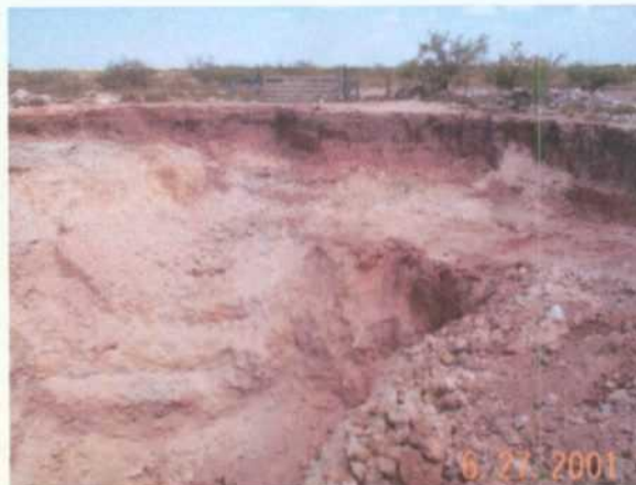
Produced water overflow pit excavation, looking SE. Depth 35 feet.
