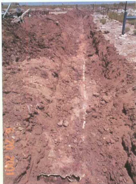
Buried PVC pipe along the east fence line that turned and headed west. Looking north.
