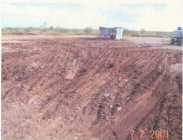
Tanks removed some contaminated soil excavated.
