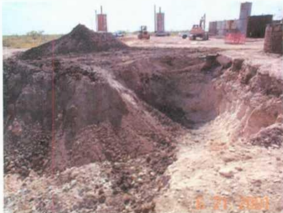
Produced water overflow pit down to 15 feet, looking west.
