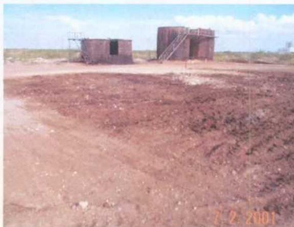
Tanks removed, some contaminated soil excavated, looking NW toward tanks 121, 111, and 112
