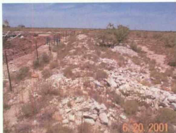
Soil/rock outside fence line to be used as clean backfill.
