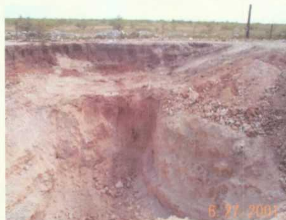
Produced water overflow pit excavation, looking south. Depth 35 feet
