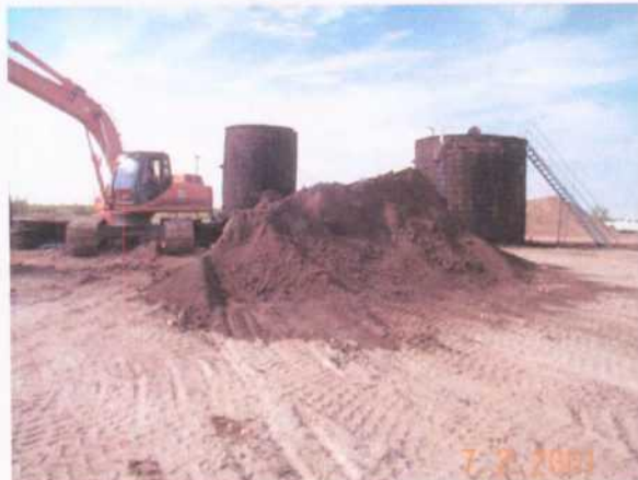
Excavation of contaminated soil and solidification of tank bottom material. Tanks 115 and 114 remaining looking south.
