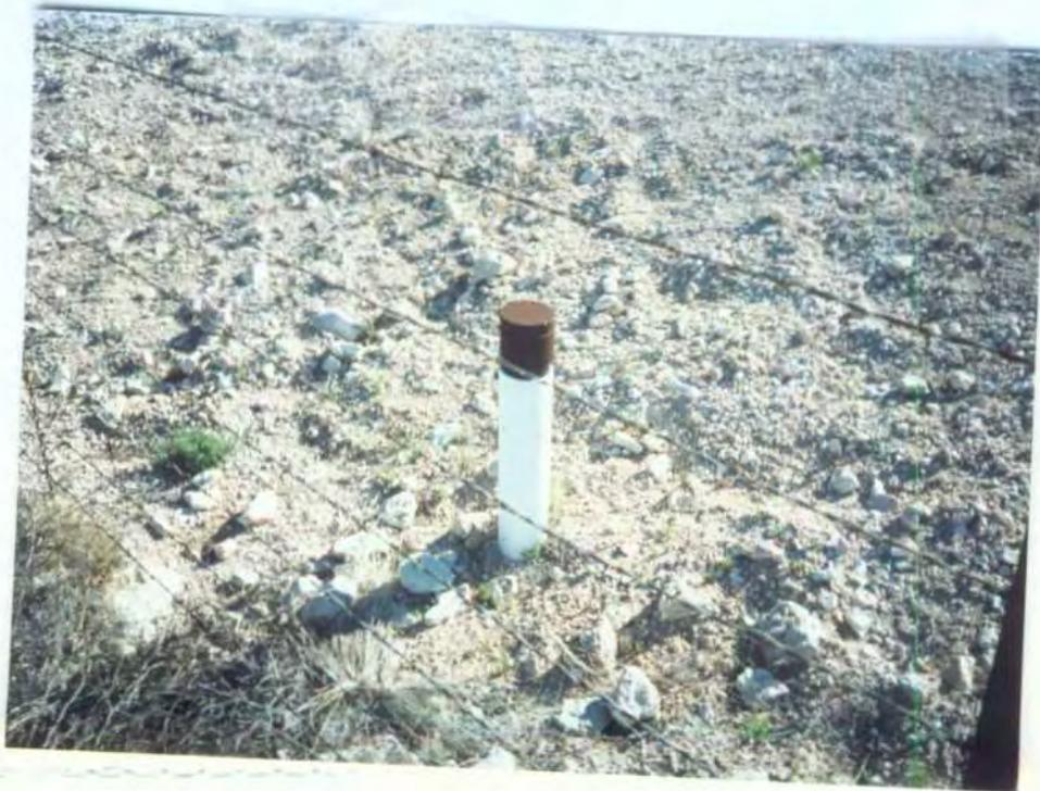
Leak Detection monitor hole
