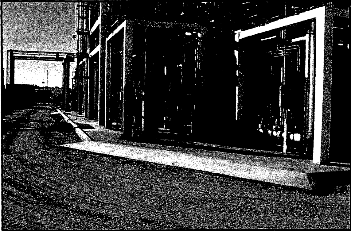
Containment Pad & Curbing – Process Area
