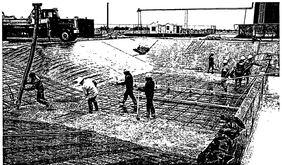
At the right edge of the photo the concrete slab is in place as the other slab is poured. Ramp with reinforcing is at the left side of photo.
