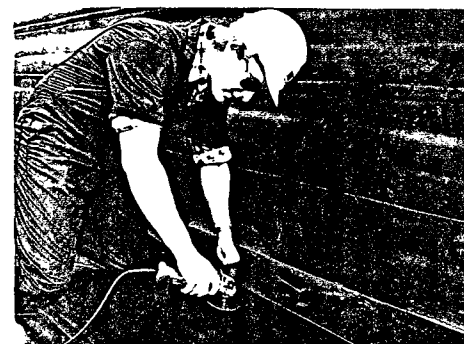
Mechanical abrasion of sheet surfaces before welding is critical to HDPE bonding.
