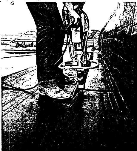
Sheets are extrusion welded using the same resin as in the sheet. This method assures a 100% integrity guaranteed seam, stronger than the sheet itself.
