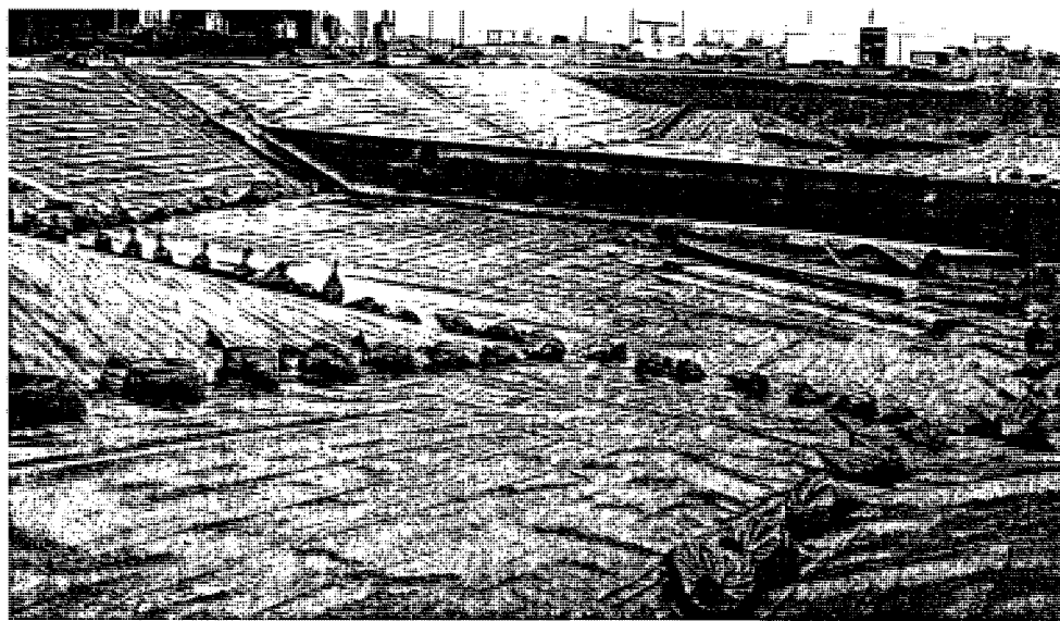
This existing pit had a concrete bottom, Gunite sides and a concrete weir. In this picture, Schlegel sheet is in place for most of the pit.
