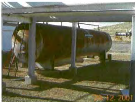
Pic#7- TEG DE-hyd knock-out tank
