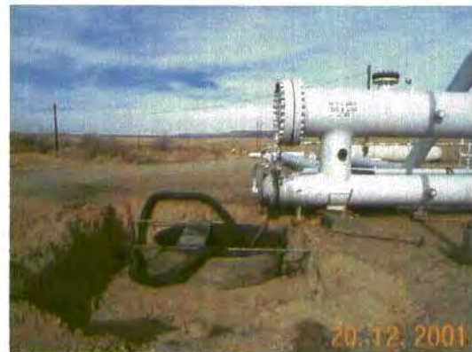
Pic#5- Main plant inlet pigging station west end.
