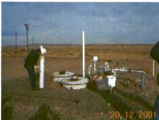
Pic#3- Main plant sump "Contact water #6" has secondary containment with Leak detection.
