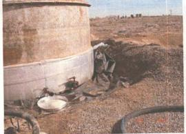
Photo 6 – Near pigging station condensate container. Disrupted liner.
