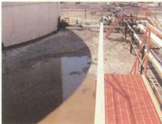
Pic #9- Water discharged from steam condensate around asphalt tanks.
