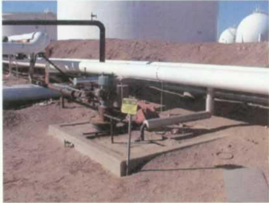
Pic #1- Main blender tank farm sump-single wall.
