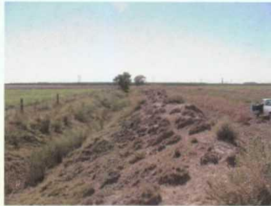
Pic #8- Standing on irrigation/drainage ditch berm looking west.
