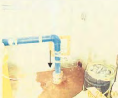
Well House #666 water sample collection point at spigot. Water flow is in direction of annotated arrow. All samples taken here were discarded, except BTEX volatiles. Reason being it was downstream of water treatment chemical injection. Chemical Pump was shut down for BTEX collection. Water well pump was running during sampling. All other samples were taken in the room next door at a petcock off of the water well line.
