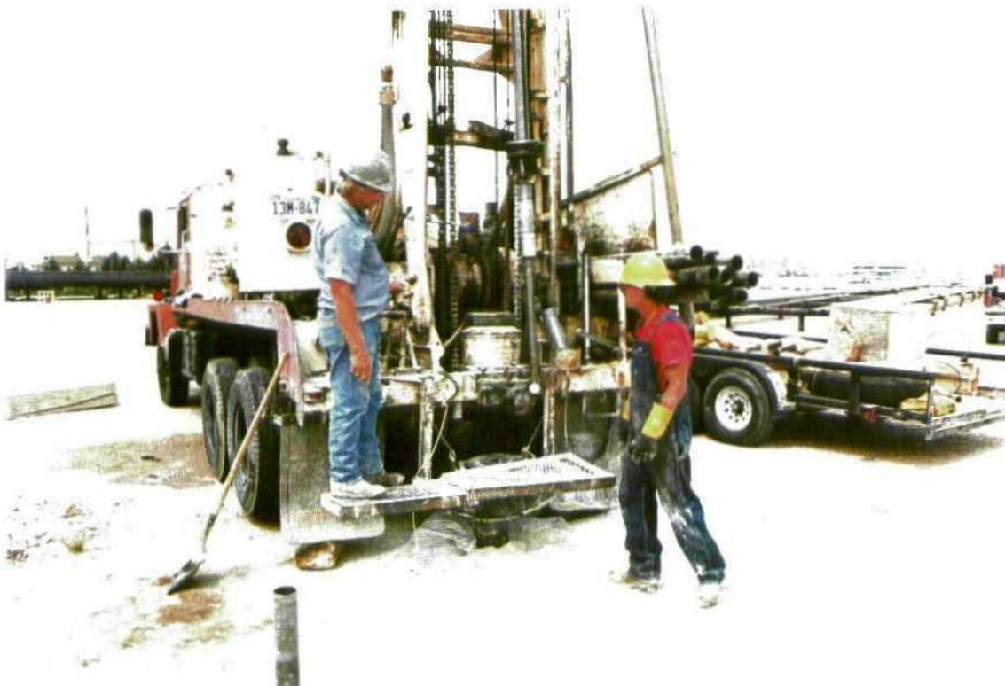
View facing northeast showing split-spoon sampling operations at monitoring well MW-5 located approximately 350 feet northwest of slop oil tank and 40 feet north of inlet gas scrubber.
