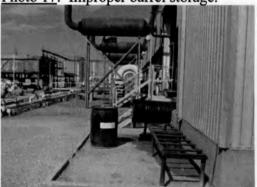
Photo 18: Improper barrel storage.
