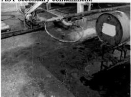
Photo 36: Discharged within unlined AST secondary containment.
