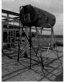
Photo 37: Unbermed/lined saddle tank.
