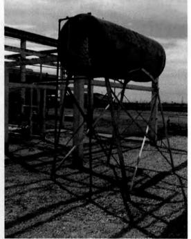
Photo 37: Unbermed/lined saddle tank.
