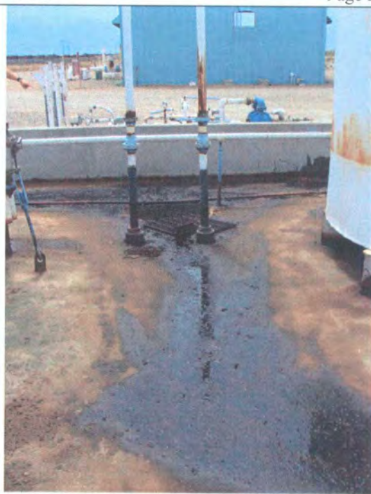
Photo 10: Fluids in secondary containment draining in to sump.
