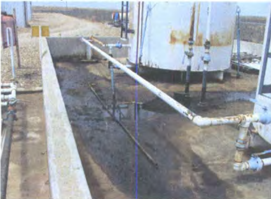
Photo 15: Fluids in secondary containment area.
