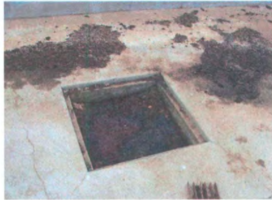
Photo 4: Sediment in sump.
