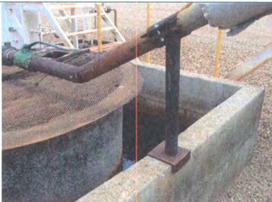
Photo 13: Fluids in secondary containment.
