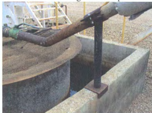
Photo 11: Fluids in secondary containment.
