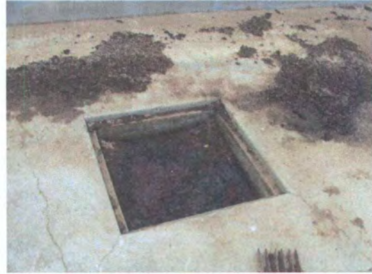
Photo 4 : Sediment in sump.
