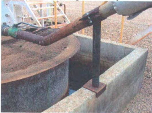
Photo 11: Fluids in secondary containment.
