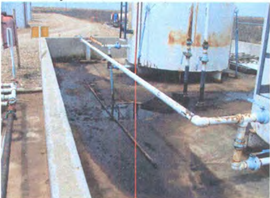
Photo 15: Fluids in secondary containment area.
