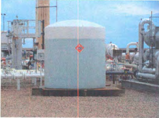
Photo 8: Un-bermed tank in processing area.
