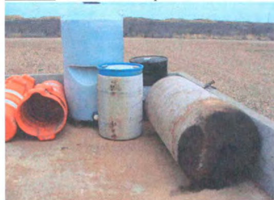
Photo 6: Containers within secondary containment.
