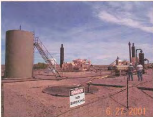
Pic # 2 wastewater tank with inlet separator below grade double wall tank.
