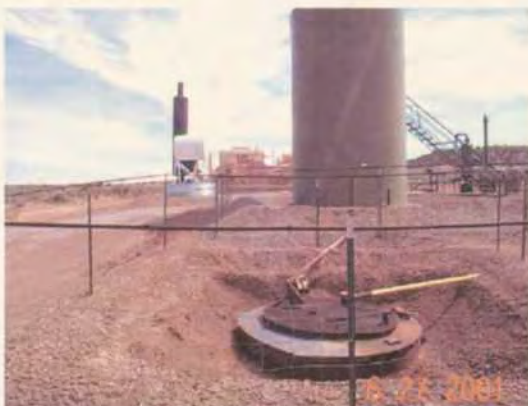
pic #3 below grade double wall wastewater tank.
