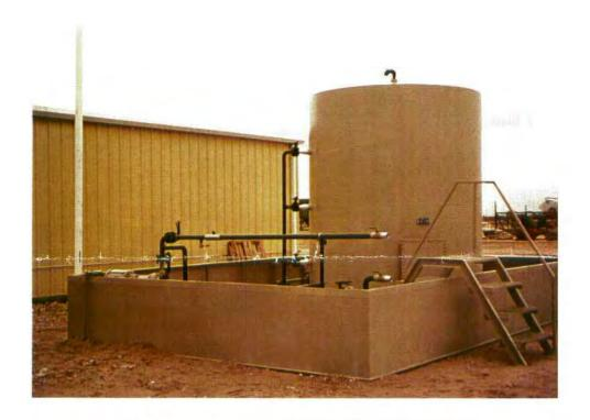
Photo 1: Diesel/Polymer Storage Vessel
