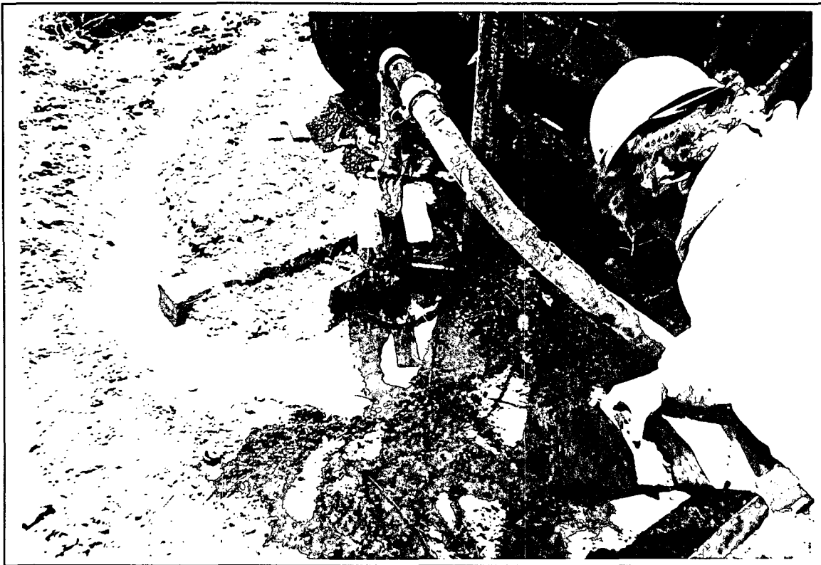
Pumping cement grout
