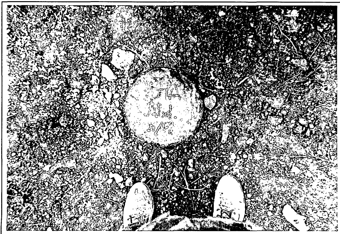
Steel abandonment cap welded to surface casing
