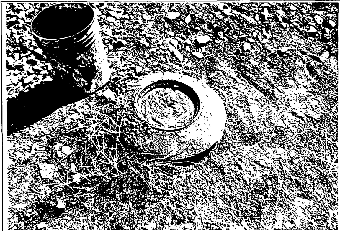
Monitor well 5-27B cement grout level at surface, prior to welding steel abandonment cap
