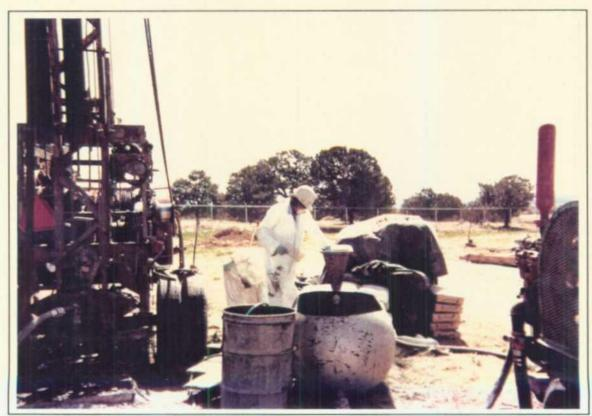
Mixing cement grout
