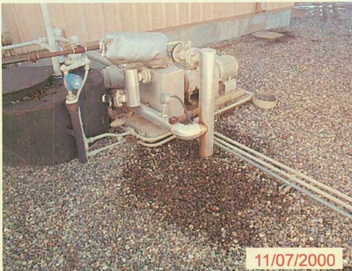
Picture #3- Oil stain near main Compressor sump pump.
