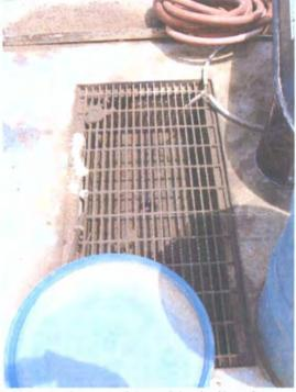
Photo 1: Sump with residual oil stains.
