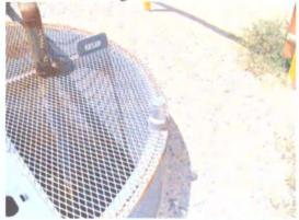
Photo 6: Leak detection port for BGT.
