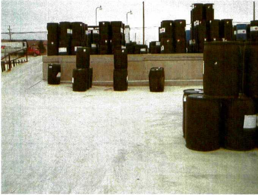
Drum storage on concrete containment area
