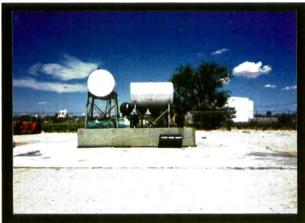
Photograph #5- View of the Bulk Chemical Storage Area identified as Area #1 on the Facility Diagram. Note the secondary containment basin and the concrete pad.
