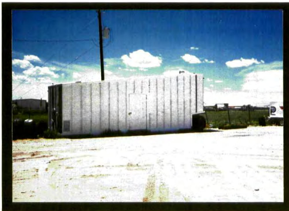
Photograph #7- View of the Chemical and Parts Storage Trailer identified as Area #4 on the Facility Diagram. The trailer is a converted 500-barrel steel construction frac tank.
