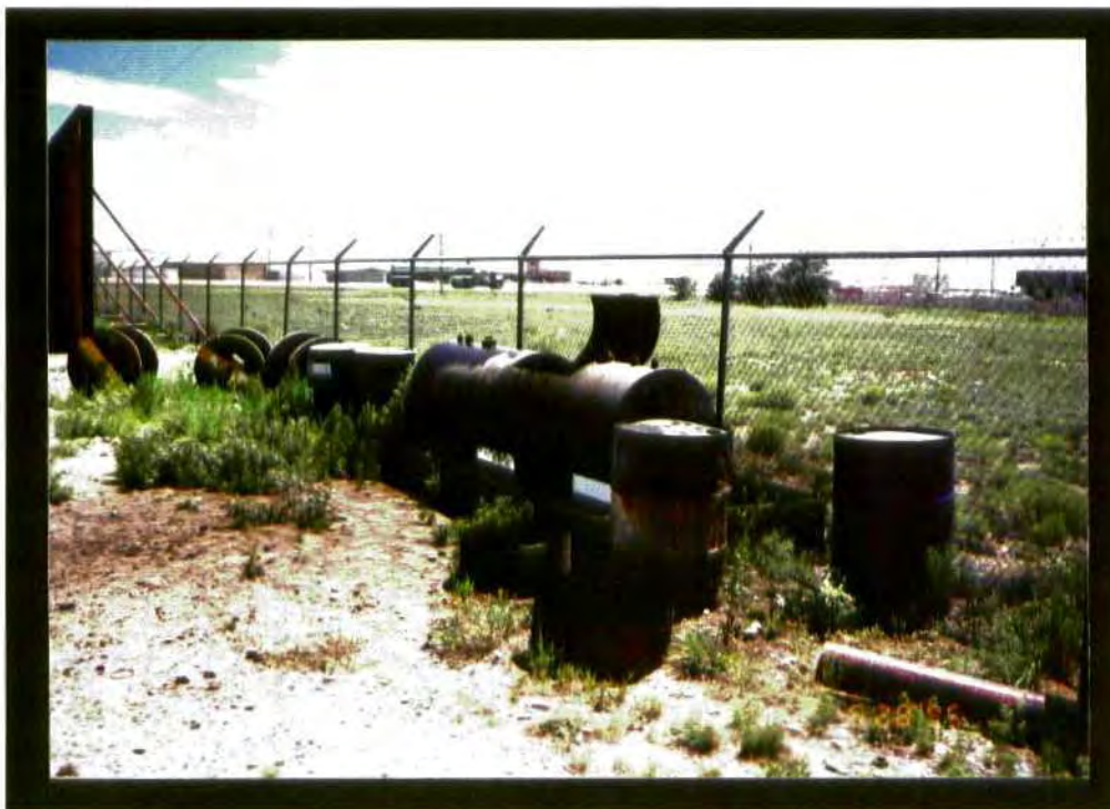
Photograph #9- View of the Waste Chemical Storage Area identified on the Facility Diagram. Note the secondary containment basin for the steel construction waste oil tank.
