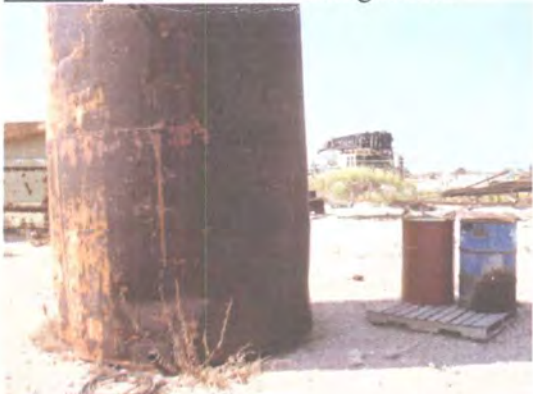
Photo 9: Tank and barrels located directly on ground no containments.
