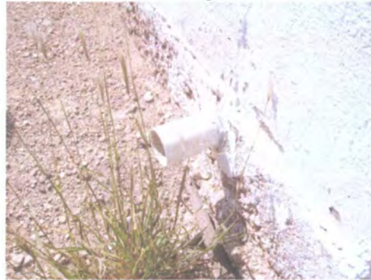
Photo 11: Cap missing on secondary containment.
