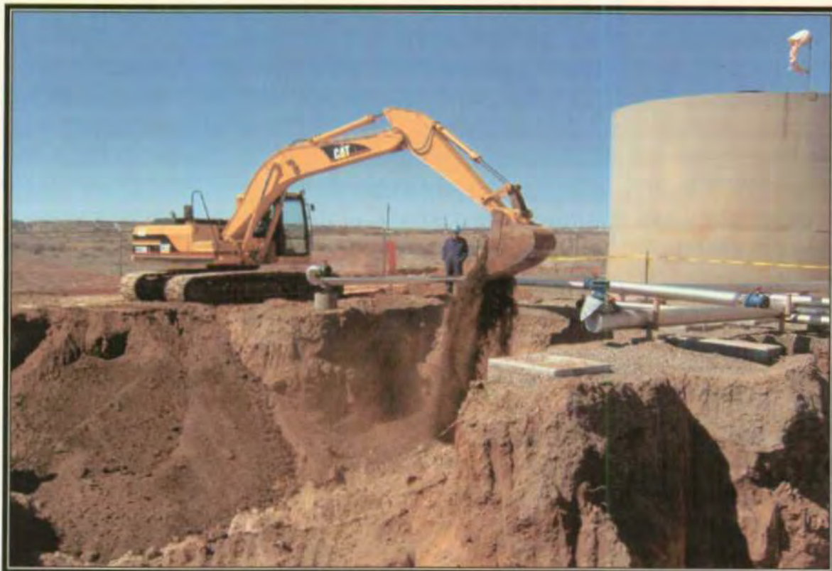
Photo 8: View of placement of the cow manure for insitu passive remediation.
