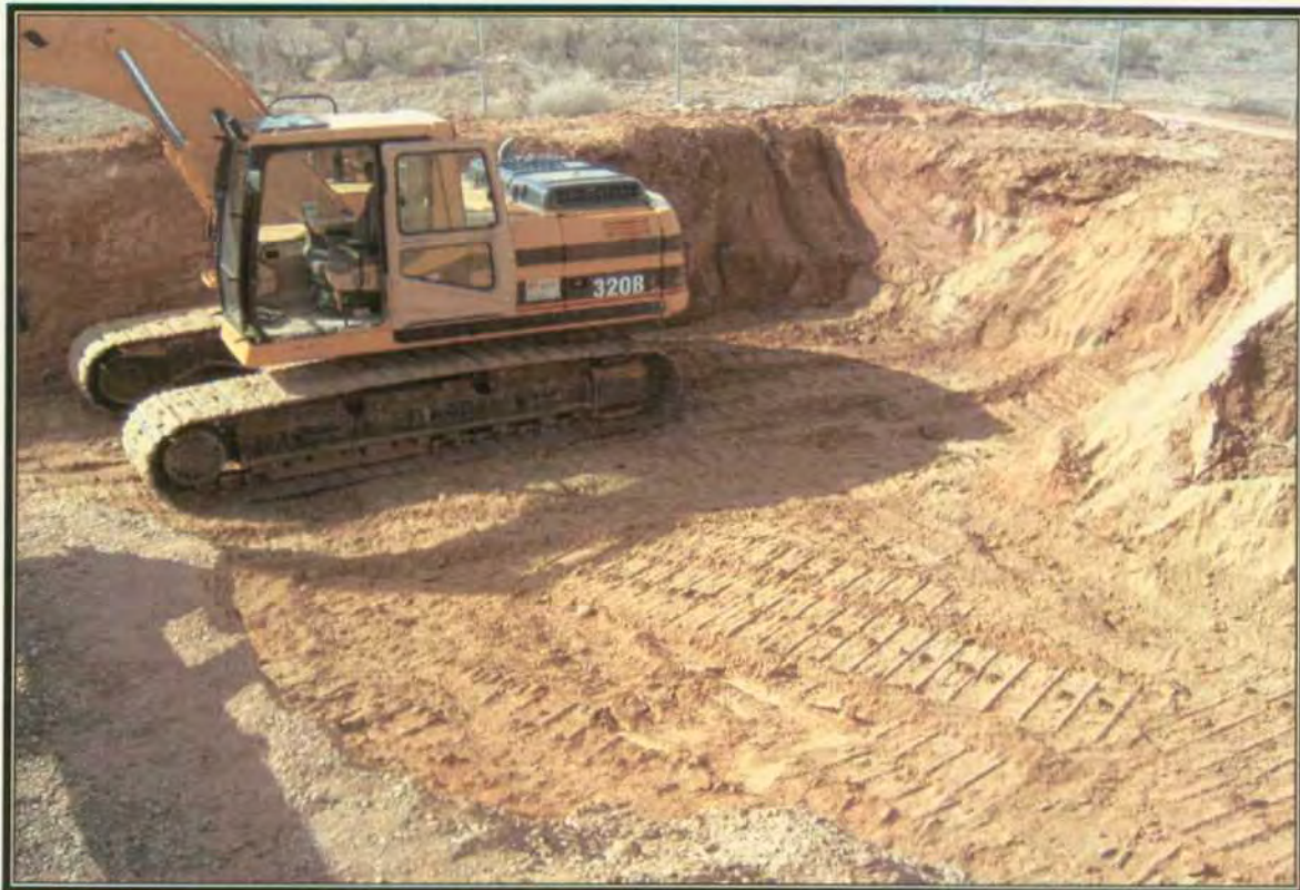
Photo 10: Continued backfill and compaction.
