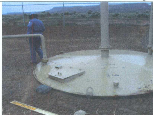
Photo 4: T411 BGT, leak detection had fluids. A rock being used as a LD cover.
