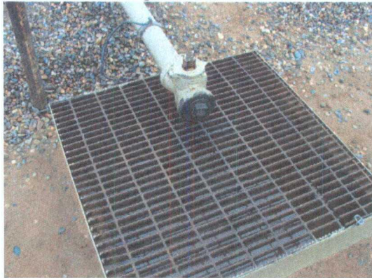
Photo 2: A secondary containment/sump with fluids. Side walls are below grade.
