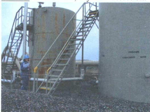
Photo 6: Unlined above ground storage tanks.
