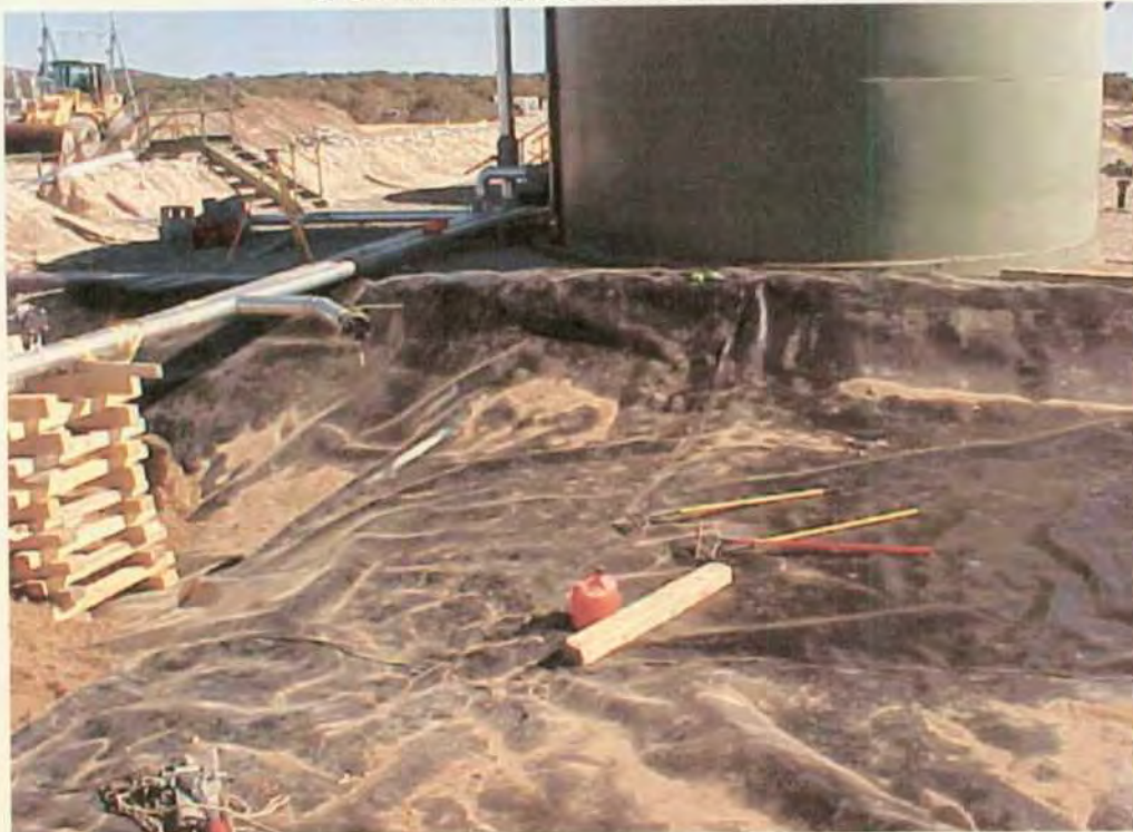
Photo 15: Installation of the HDPE liner. The liner overlapped the existing berms and the newly constructed small berm, seen in the middle of the photo. Photo taken looking to the east.
