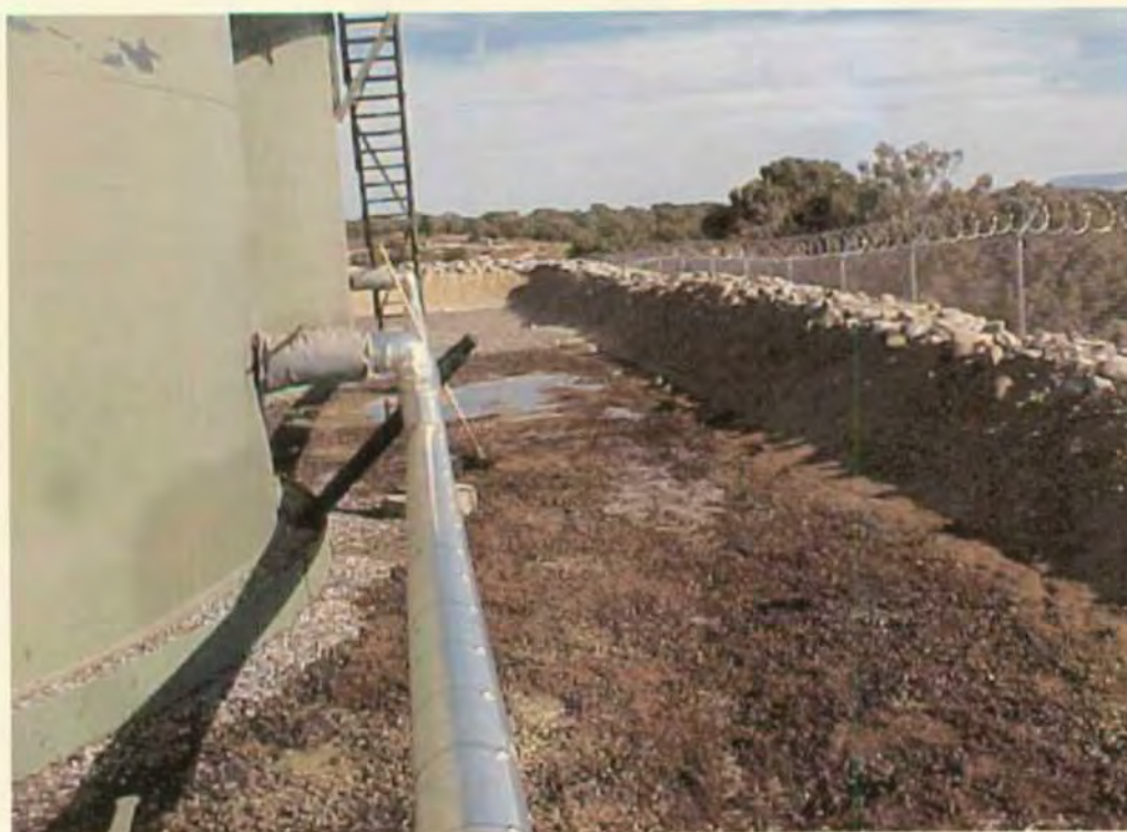
Photo 6: Environmental absorbant material was spread over the remaining standing liquid. Photo taken looking to the east.
