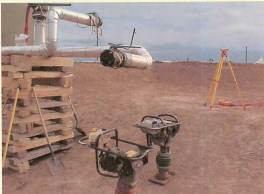
Photo 14: Compaction of the native soil to prepare for the installation of the HDPE liner. The live lines were capped and cribbed in place. Photo taken looking to the south.
