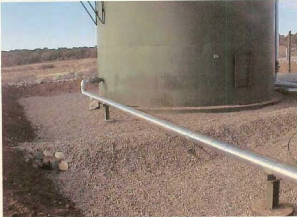
Photo 19: Completion of the site restoration. Overflow pipe in the small berm can be seen in the lower left hand corner of the photo. Photo taken looking to the west.
