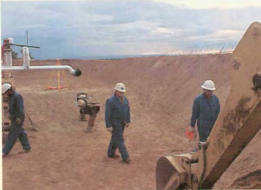
Photo 13: Compaction of the native soil to prepare for the installation of the HDPE liner. Liner design, shallow to deep, can be seen in this photo. Photo taken looking to the south.
