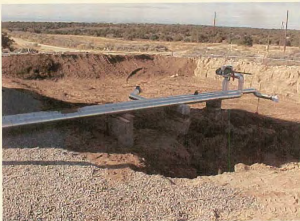
Photo 12: Site after the removal of the western most tank, "sump", and contaminated soil. The live pipes in the foreground are cribbed. Photo taken looking to the southwest.
