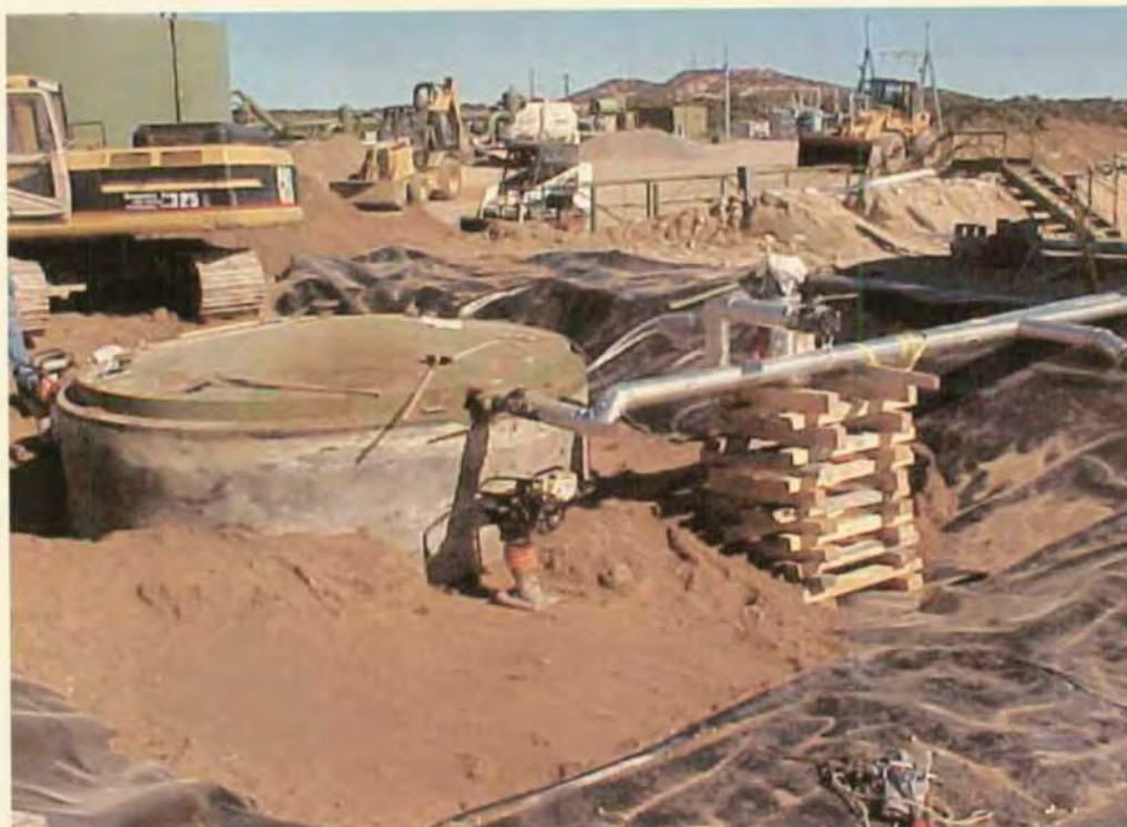
Photo 16: Aggregate Base Coarse was compacted around the sump. Photo taken looking to the northeast.
