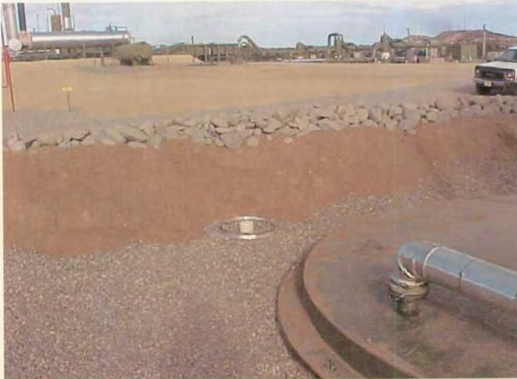
Photo 21: Completion of site. 18" corrugated metal pipe with 4" PVC pipe to facilitate in the removal of product if another spill occurs. Photo taken looking to the northeast.
