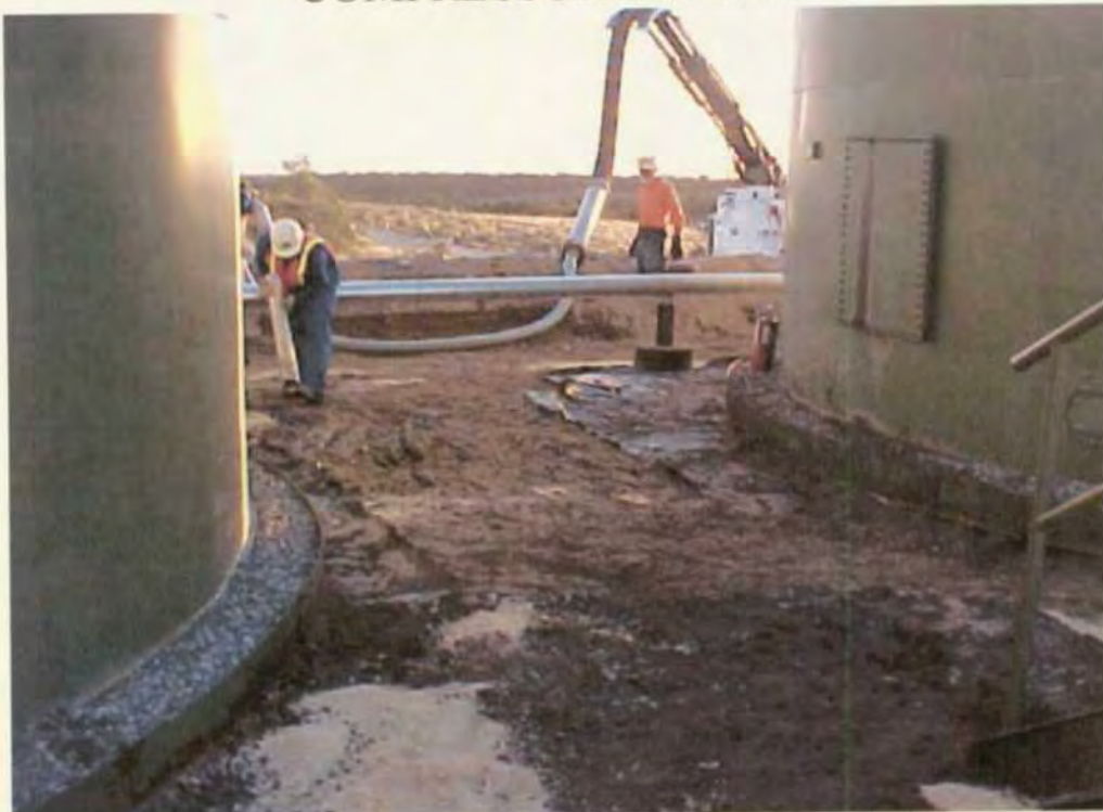
Photo 7: Badger Daylighting Corporation truck vacuum excavating the contaminated soil. Photo taken looking to the south between the two western most tanks.
