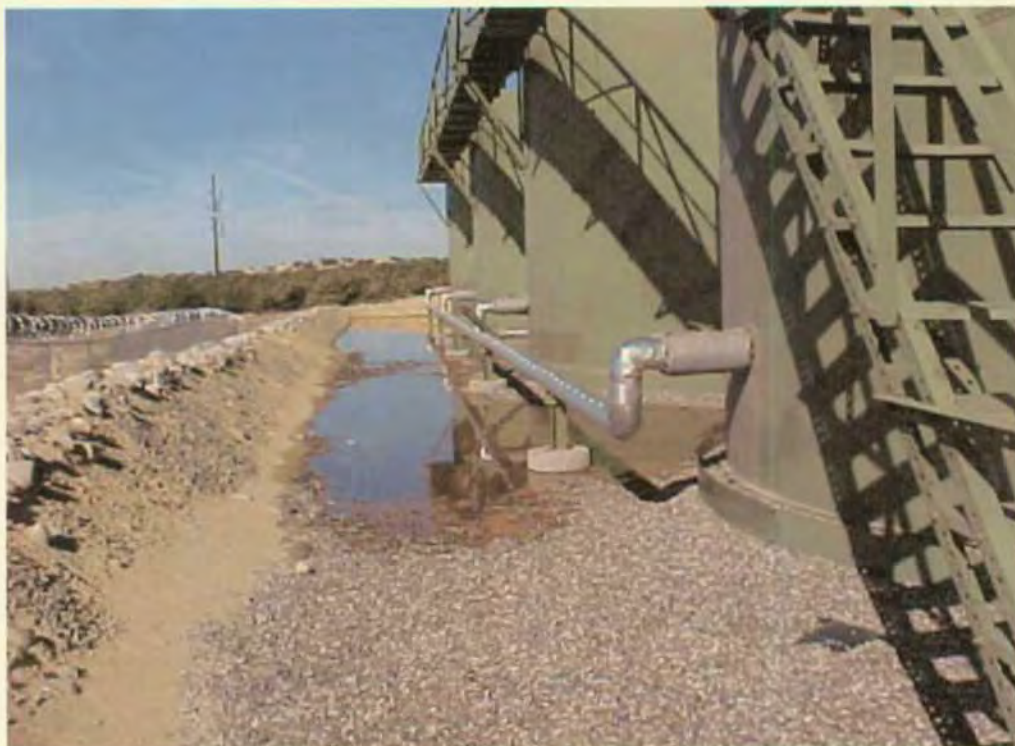
Photo 2: Spill along the southern boundary of the secondary containment. Photo taken looking to the west.
