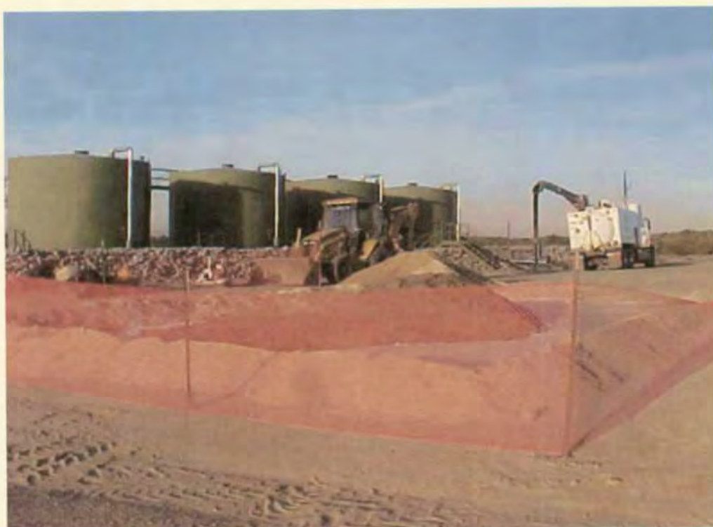
Photo 8: Contaminated soil stockpile on site. Photo taken looking to the southwest.
