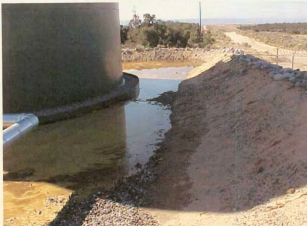
Photo 3: Spill along the western boundary of the secondary containment. Photo taken looking to the south.
