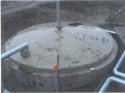
Photo 1: 1 BGT (T207) verified DRY leak detection system.
