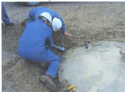
Photo 3: BGT (206) verified fluids in leak detection system.
