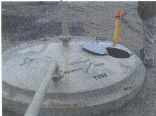
Photo 2: 2 BGT (T208) verified DRY leak detection system.
