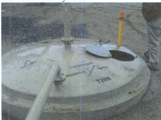
Photo 2: 2 BGT (T208) verified DRY leak detection system.
