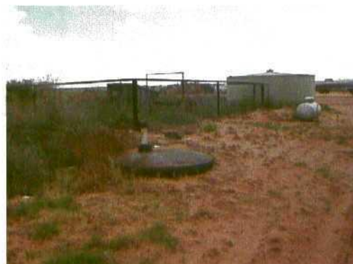
old below-grade tank-not used, has no secondary containment.
