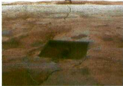
Wash bay sump-looking east sump drains to below grade tank shown in background. Below-grade tank does not have secondary containment.
