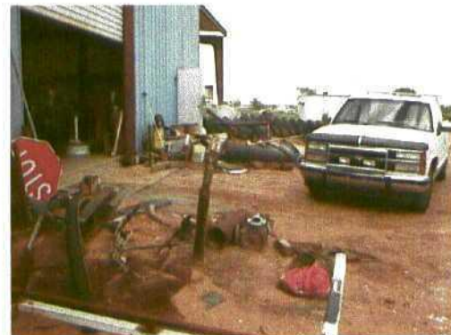
Below-grade waste oil tank drain pipe sticking up from tank. Tank has no secondary containment.
