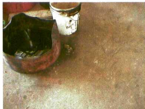
Floor drain for waste oil goes to below-grade waste oil tank.
