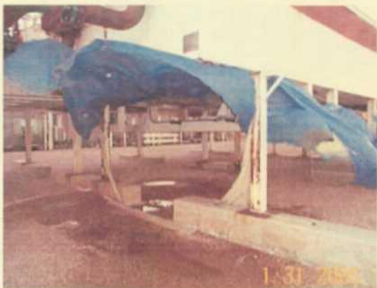
Fin-fan water leak
