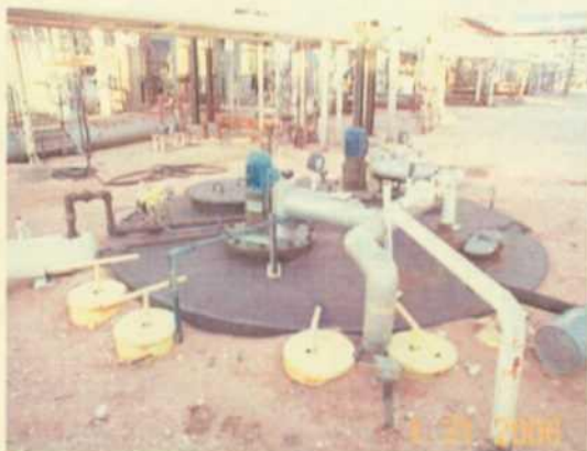
New Plant Sump with secondary containment.
