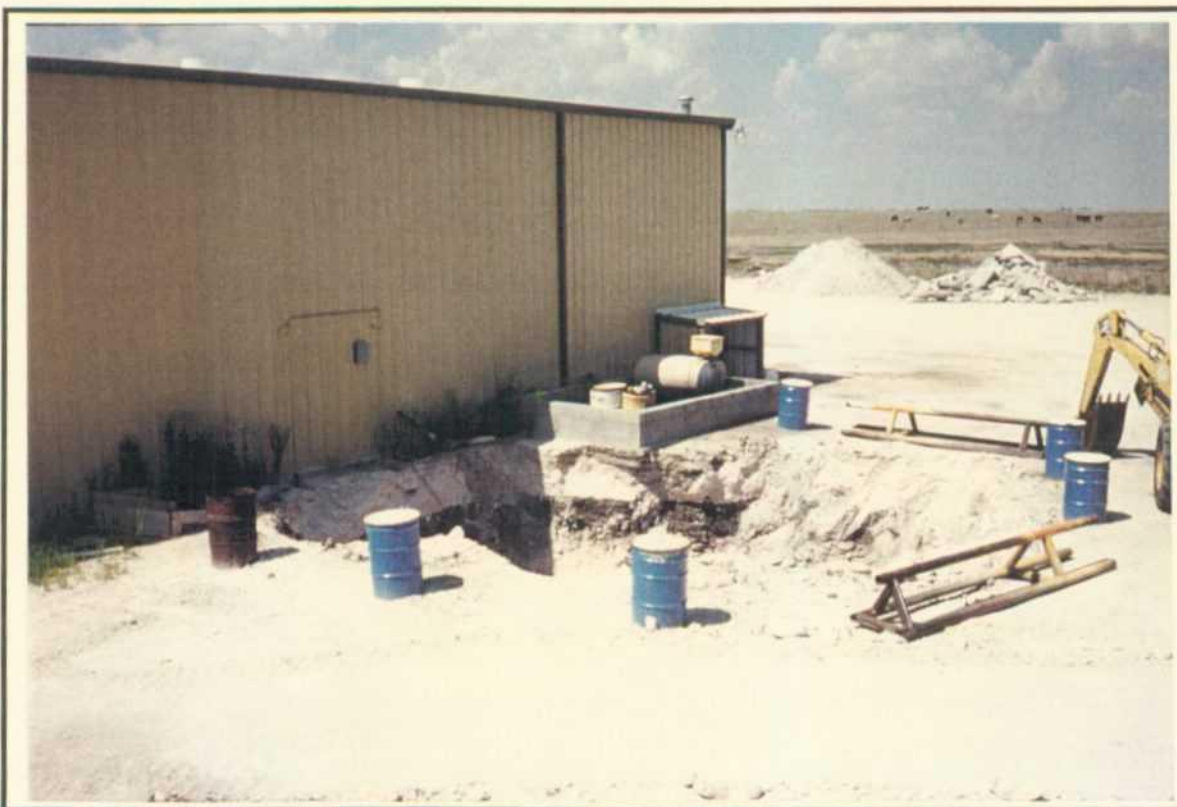
Photo 32: Final excavation limits of mechanics pit/leach field.
