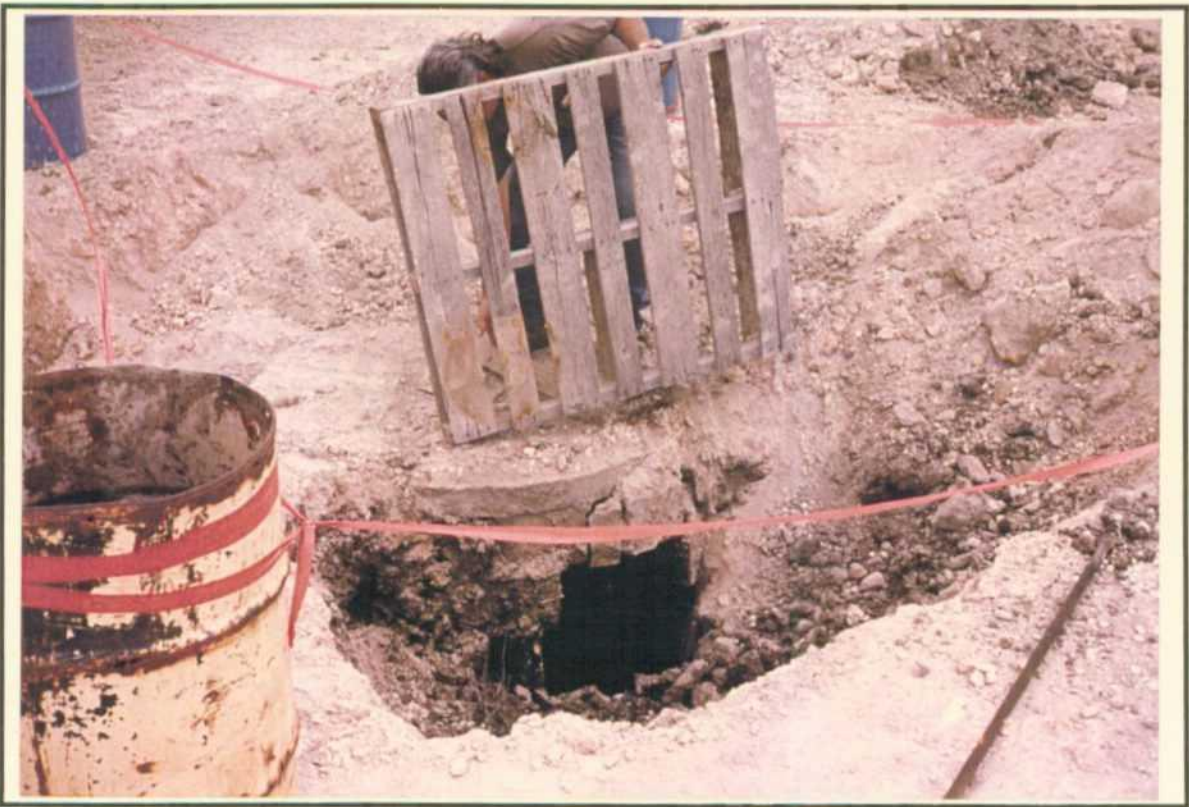
Photo 16: Northeast wash bay seepage pit exposed.
