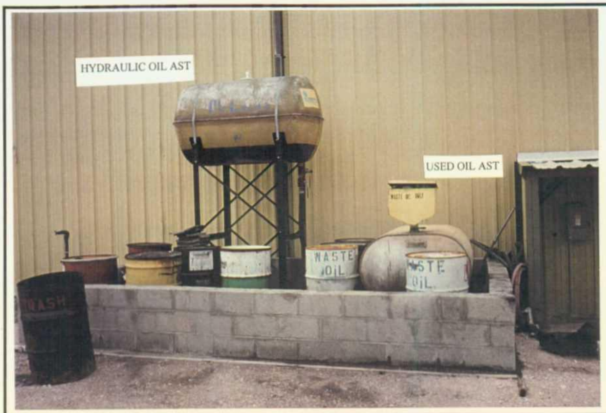
Photo 5: Hydraulic and used oil AST area with containment.
