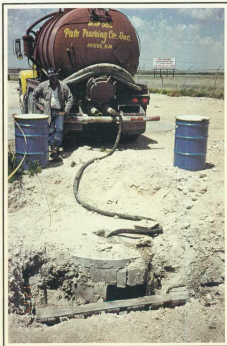
Photo 18: Fluids removal from wash bay seepage pit.
