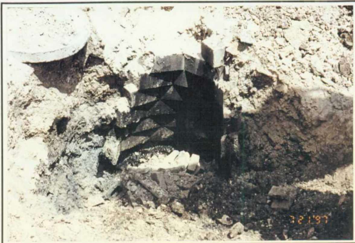
Photo 29: Typical concrete block constructed seepage pit.
