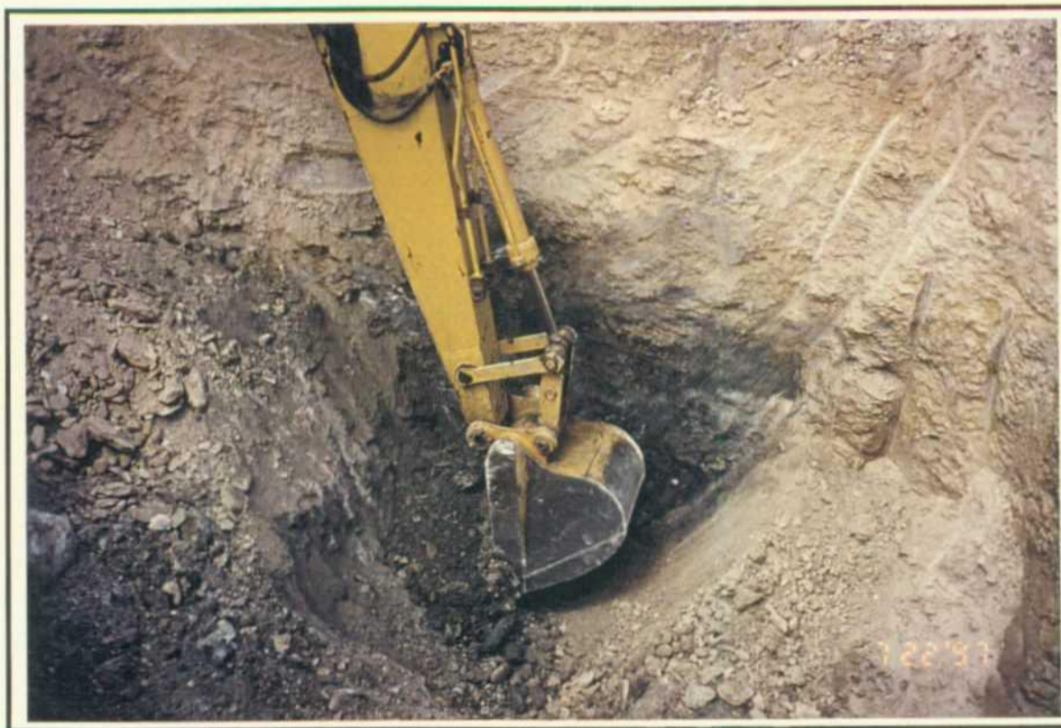
Photo 30: Impacted soil contact at mechanics pit/leach field.
