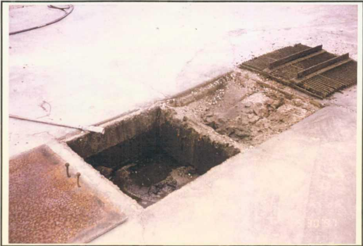
Photo 15: Wash pad drain location. Note Northern sump is near total capacity with solids.
