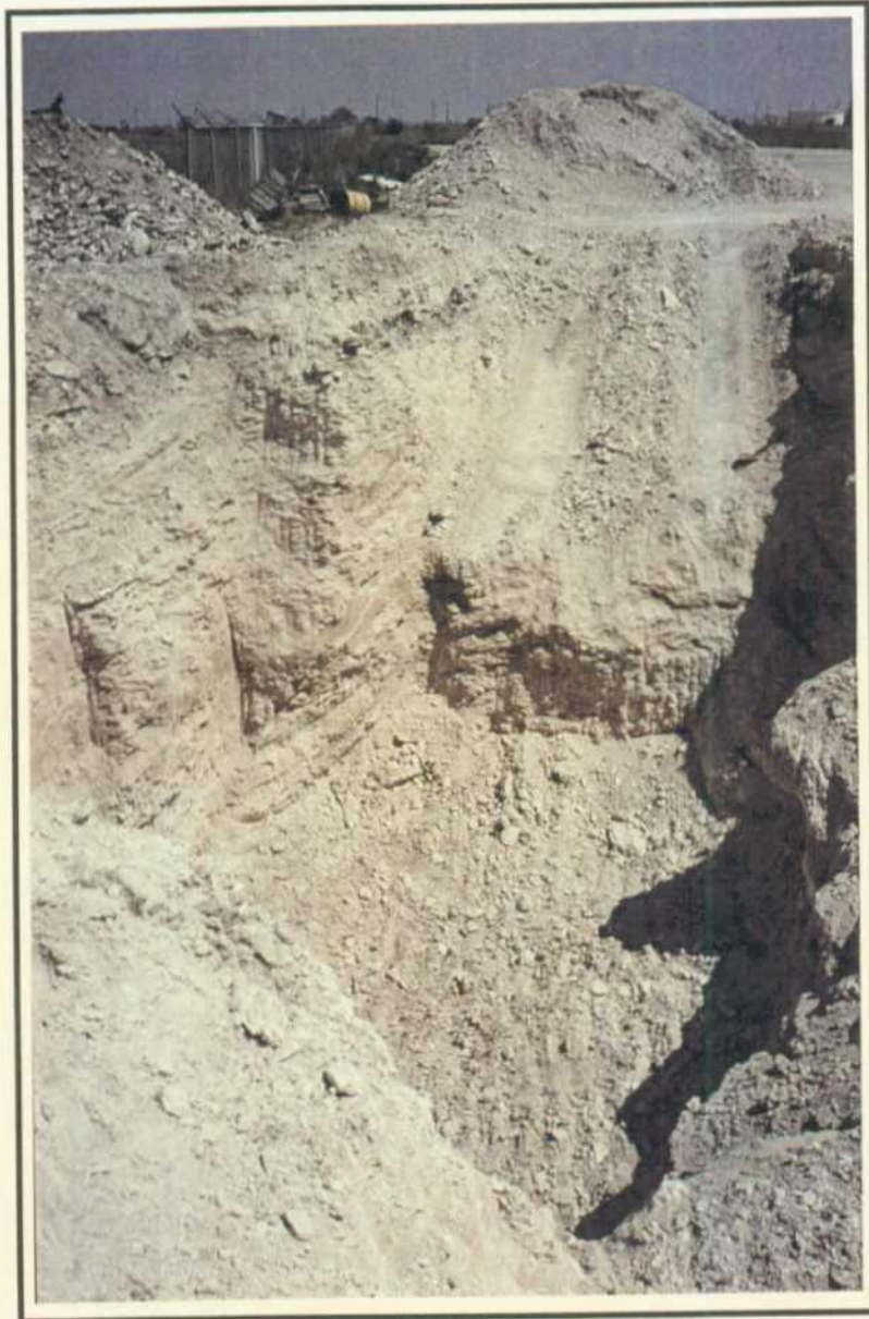
Photo 23: View South of Northeast wash bay excavation. Note Floor area excavated to 21 feet below ground level.
