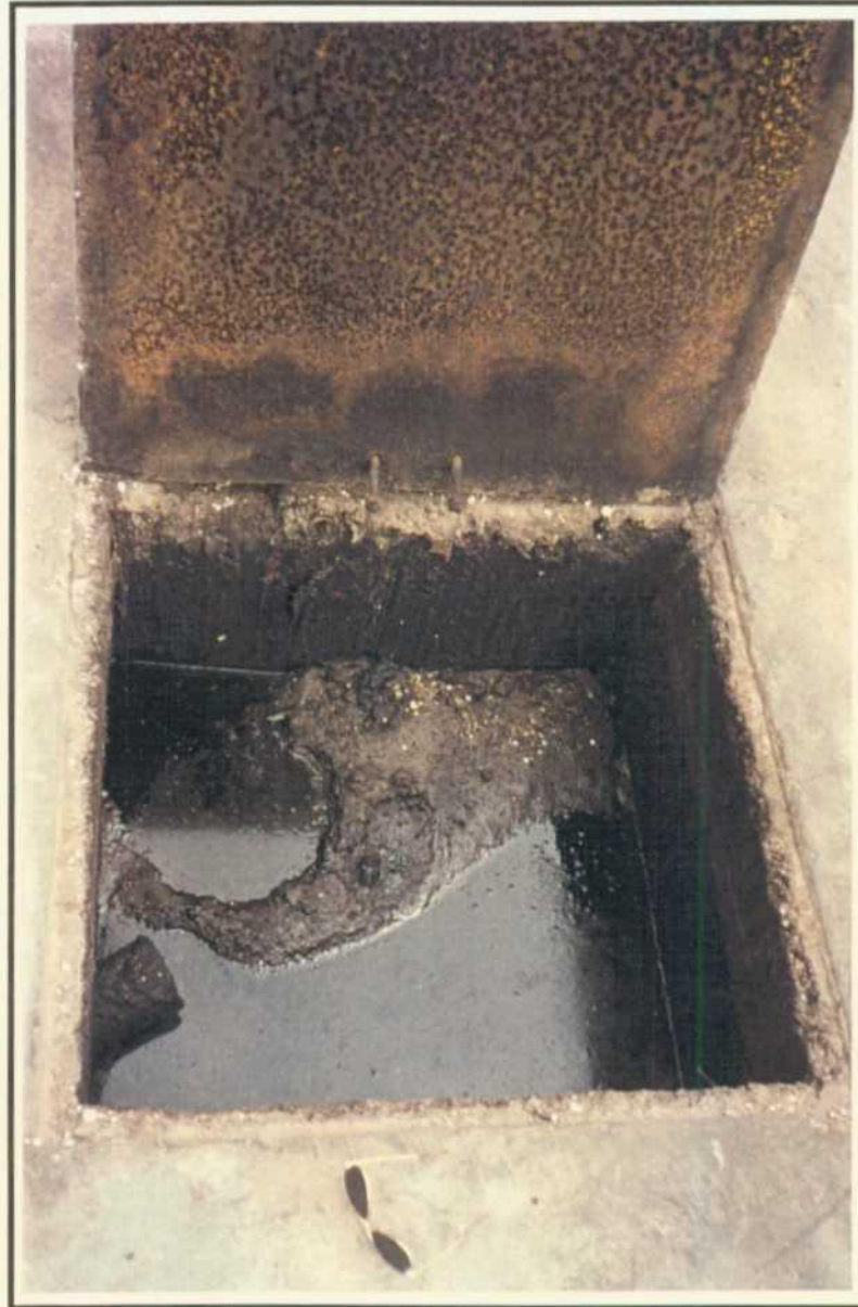
Photo 17: Wash bay drain/sump with fluids and solids.
