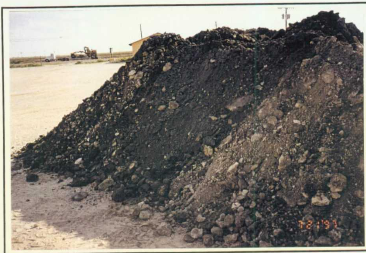
Photo 21: Typical impacted soil excavated from Northeast wash bay/seepage pit.
