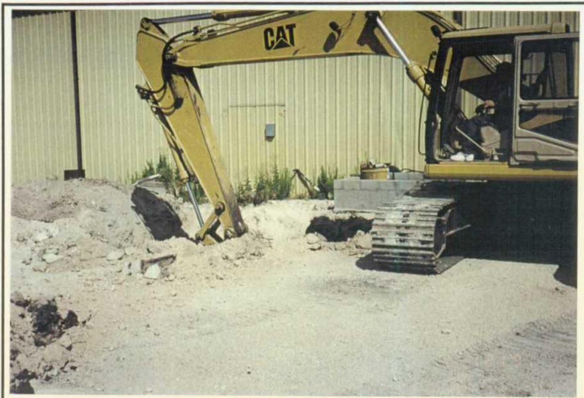
Photo 26: Excavation of surface cover above leach field.
