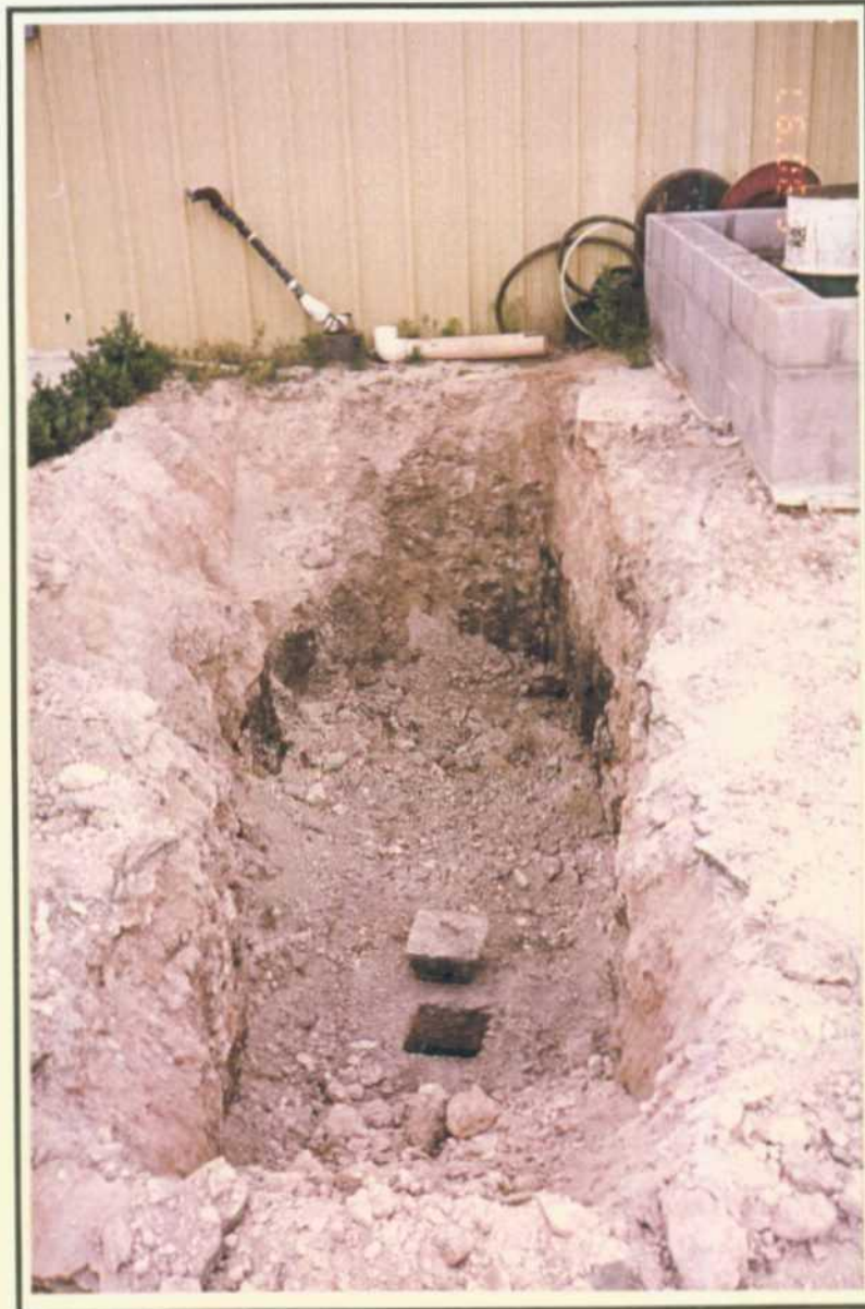
Photo 28: Mechanics pit uncovered. Note access piping port.
