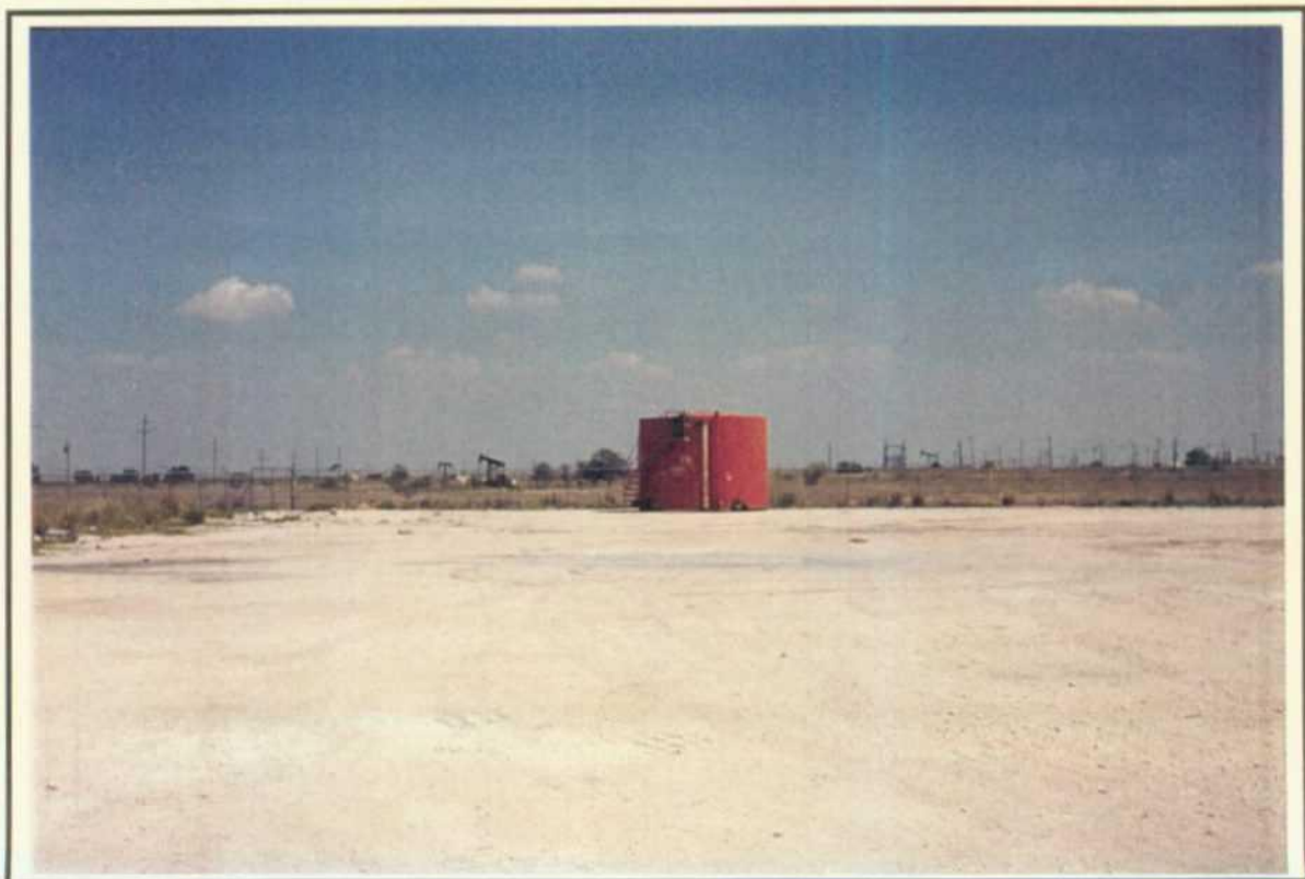
Photo 12: Temporary storage tank (frac tank) for fluids removed from seepage pits.
