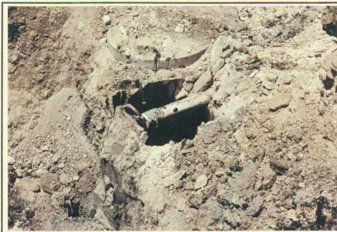
Photo 27: Drain line entering mechanics pit/leach field.
