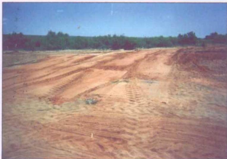
Backfilled With Clean Topsoil
