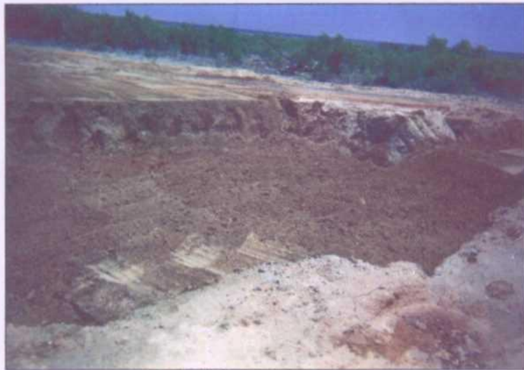
Backfilled to 4 ft; Before Liner
