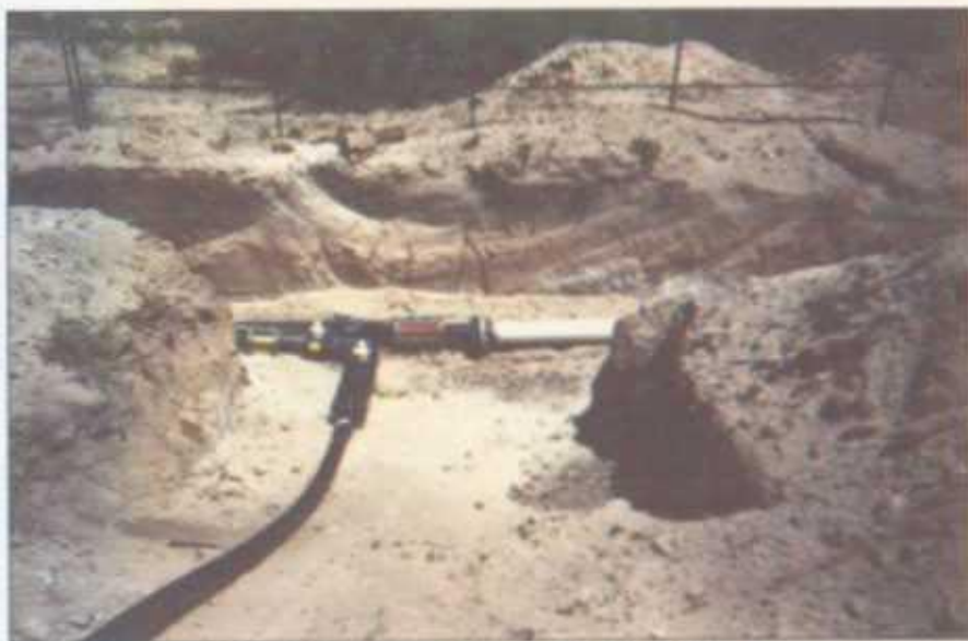
New Plumbing At New Jct. 90 ft West
