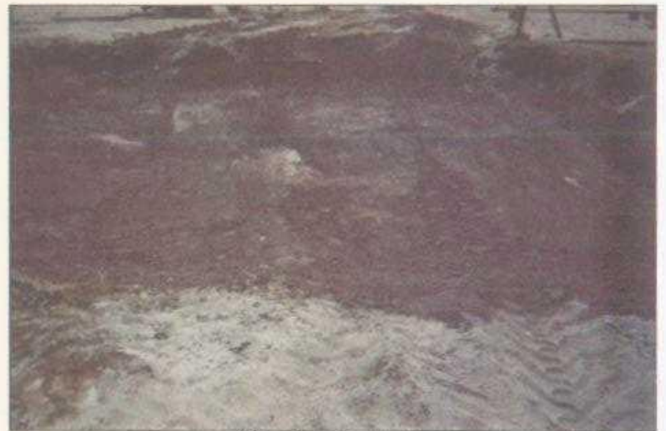
Clay Barrier At 4 ft
