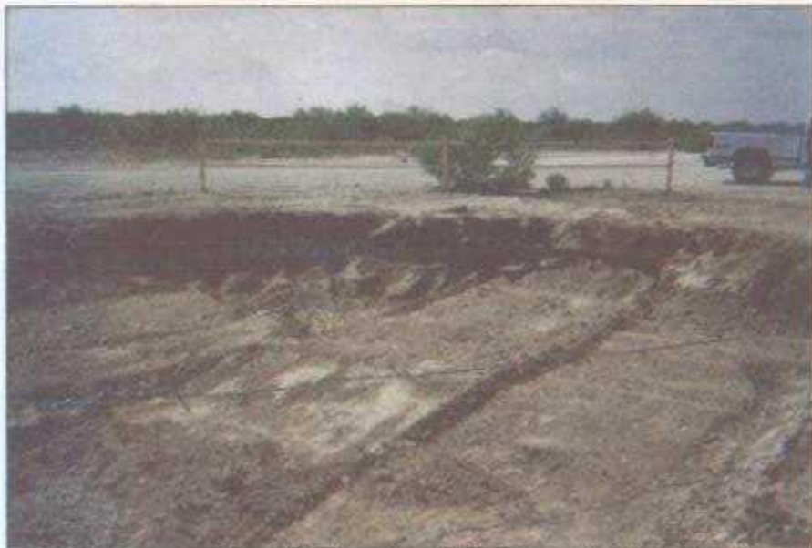
Excavation Backfilled to 4 ft With Remediated Backfill
