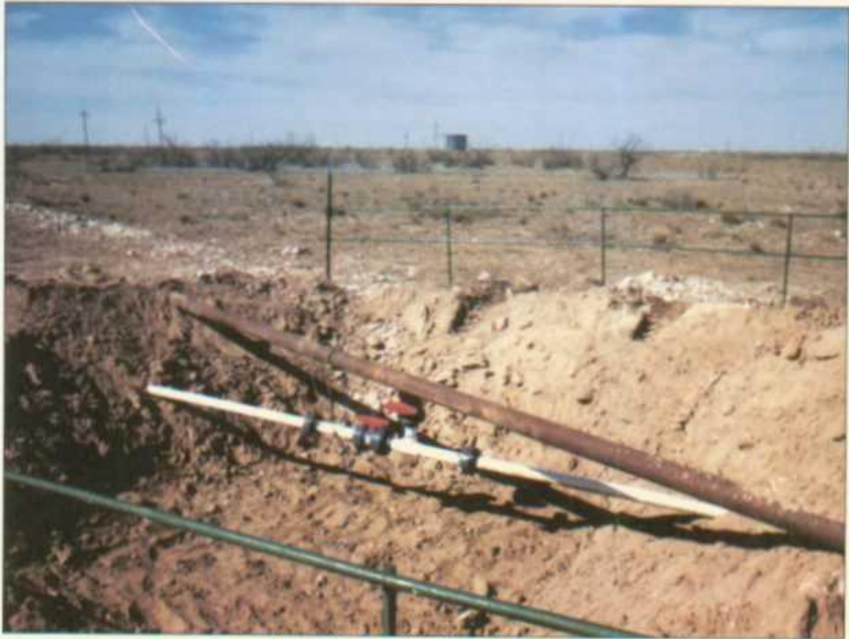
Remediation with New Plumbing
