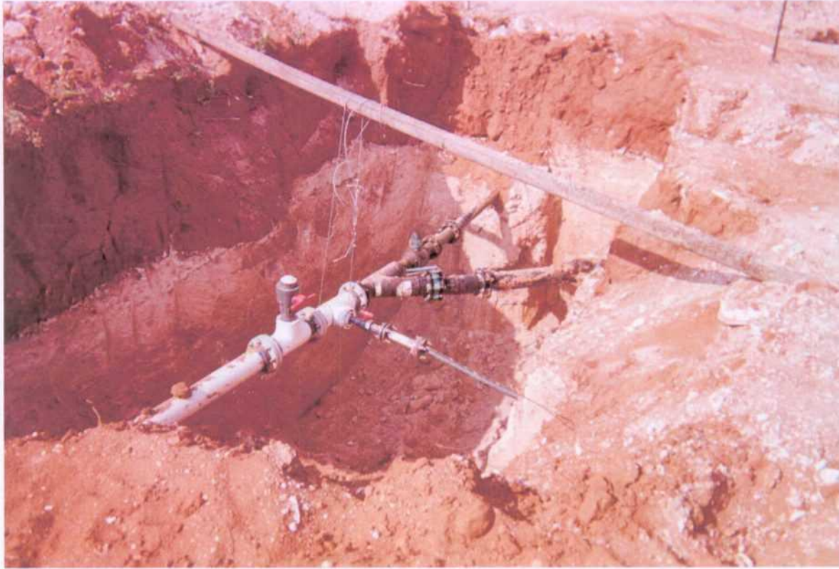
Impact excavation from new jct. O-17
