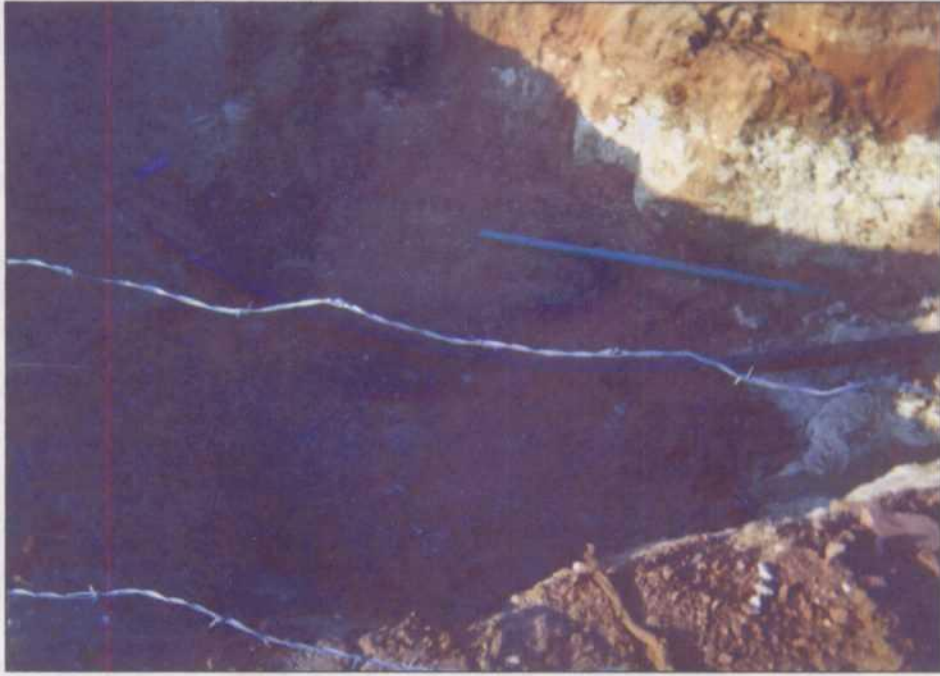
Compacted Clay Barrier
