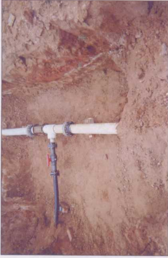
new plumbing for new junction 25 ft South
