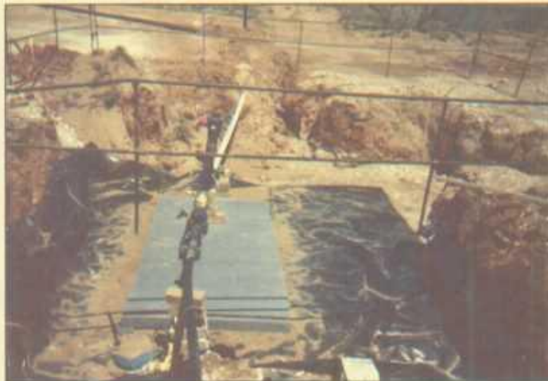
Box Construction (with poly liner)
