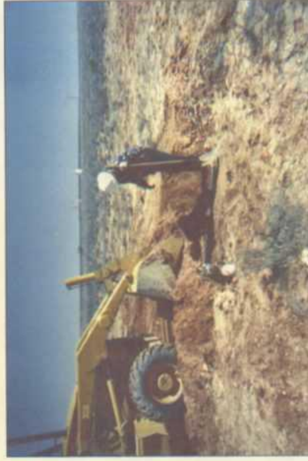
Backfilling excavation
