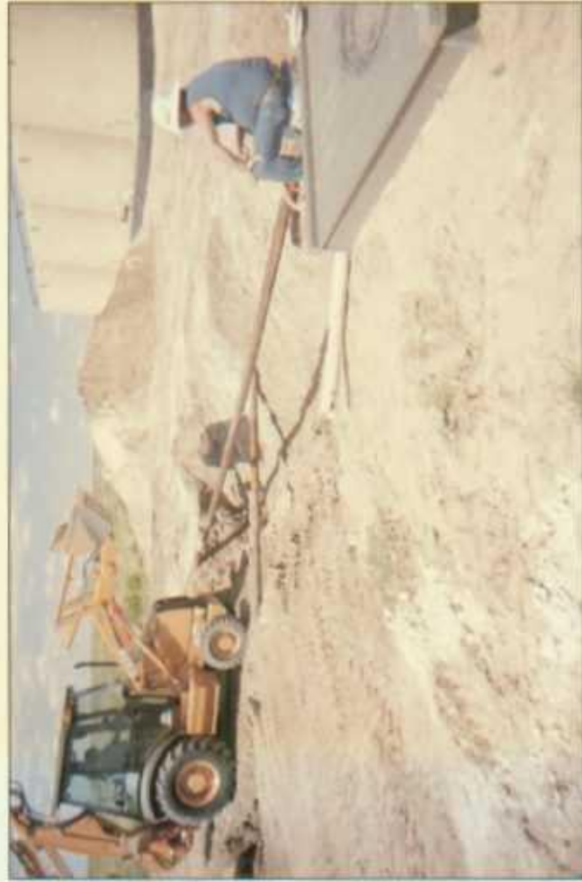
backfilling excavation (with new junction box)
