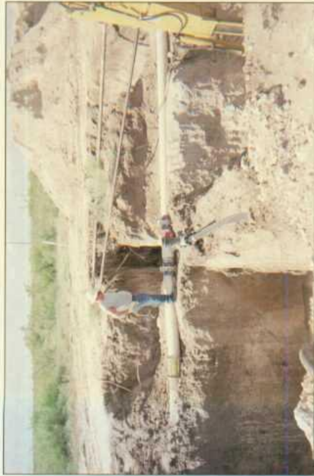
30 x 30 x 12-ft excavation with pipe supports
