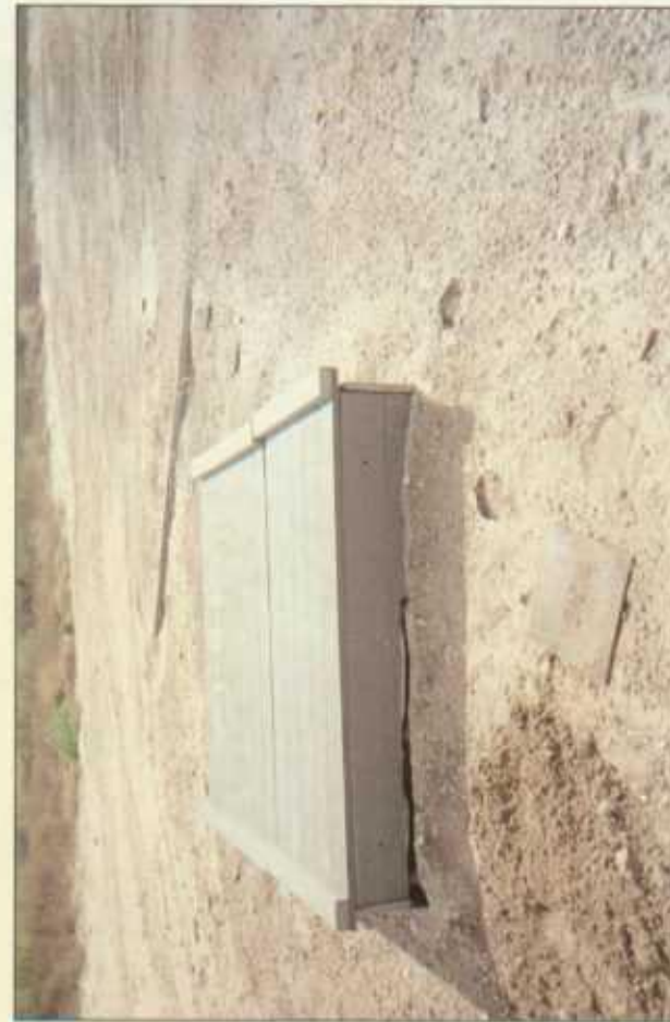
disclosure plate at junction box
