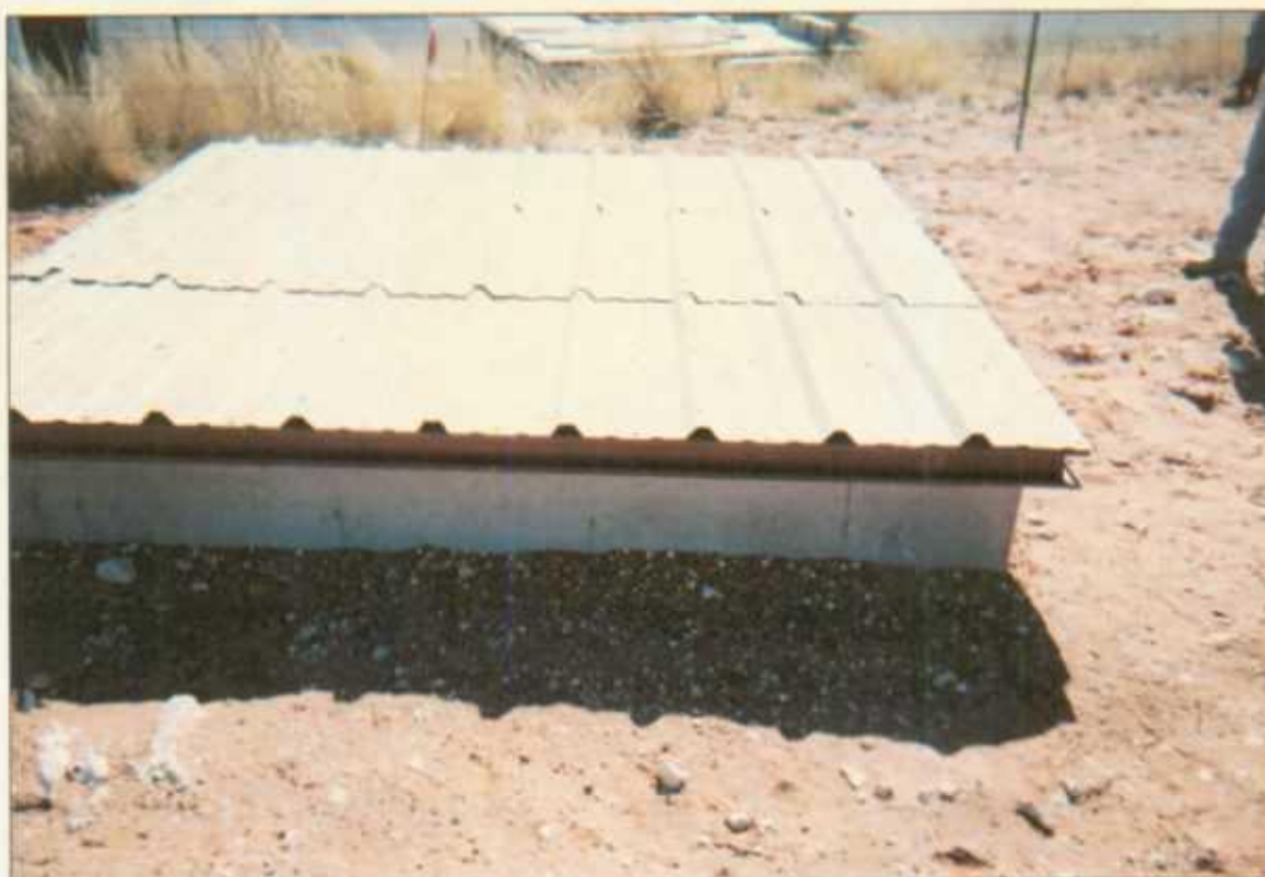
new watertight junction box 5 ft southeast of former box
