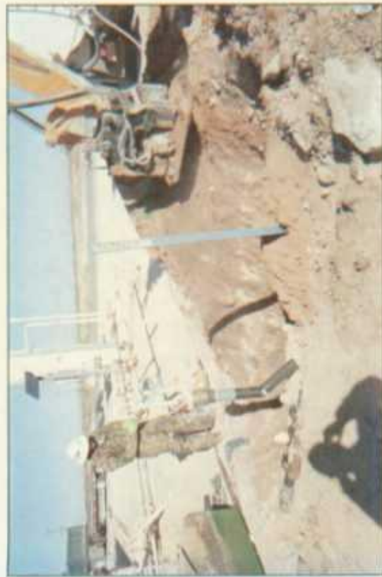
backfilling trench
