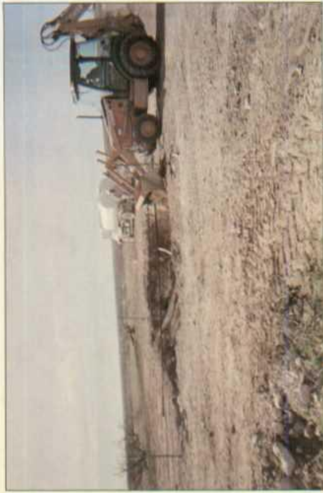
backfilling excavation
