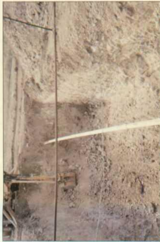
completing 10 x 20 x 12-ft-deep excavation
