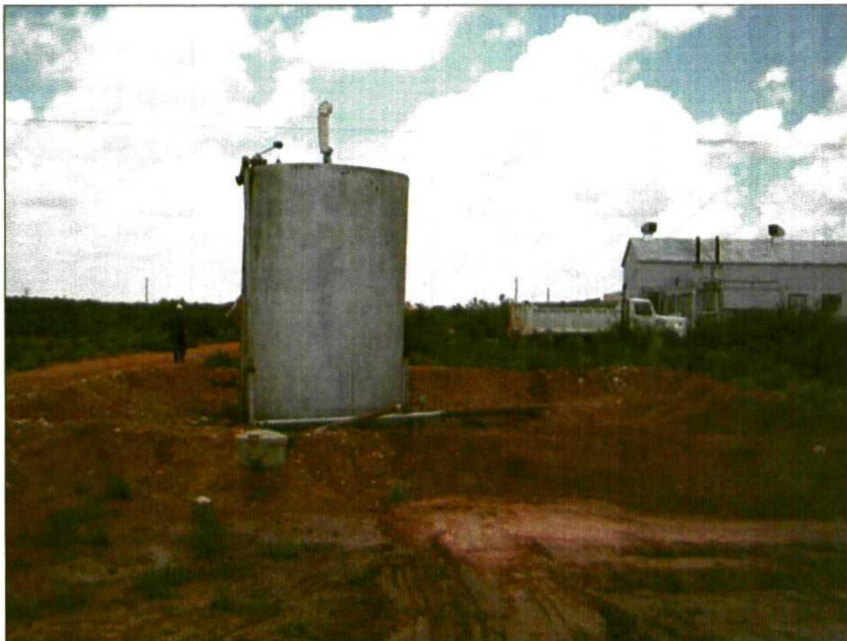
FIGURE 2. Lusk Compressor Station Slop Oil Tank (40' x 40')
