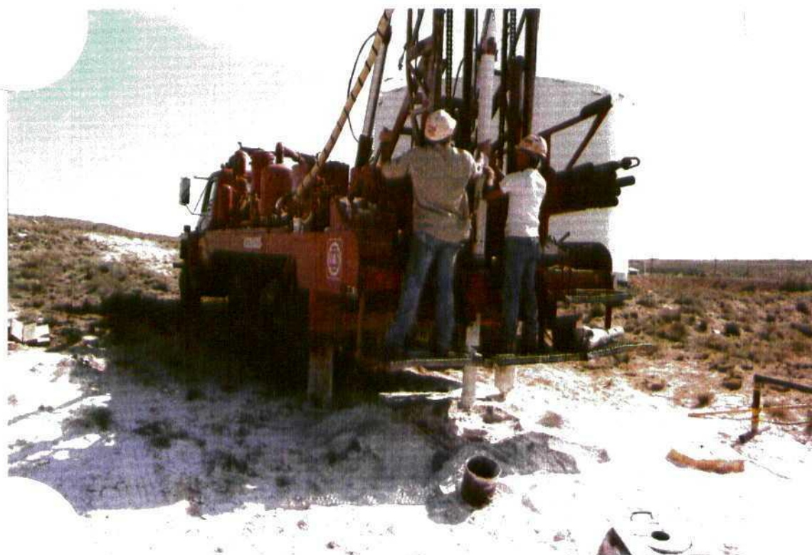
Photograph 4: View of monitor well screening operations for MW-2.
