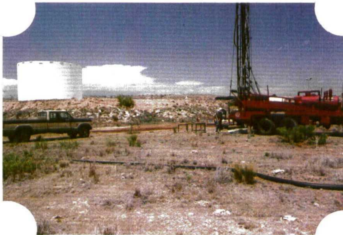
Photograph 5: View looking northwest showing drilling operations for MW-1 located in Scoggin Draw near the southeast corner of the site.
