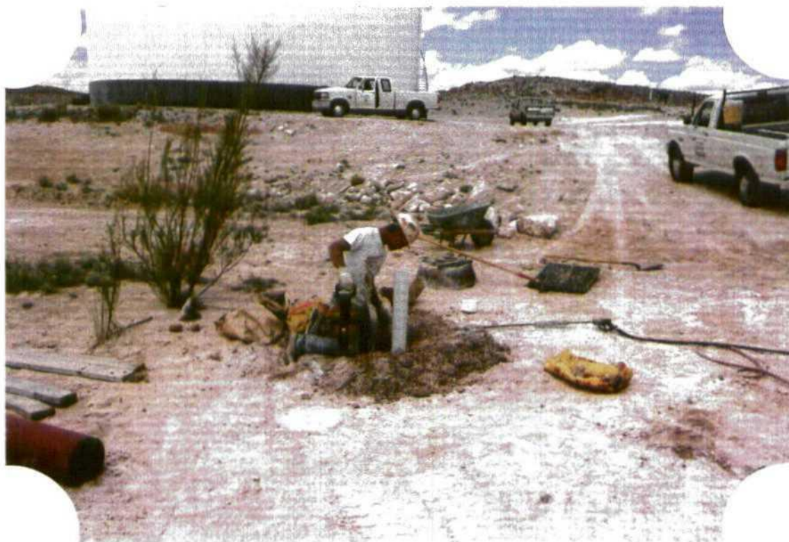
Photograph 6: View of well completion operations (bentonite seal) for MW-3 located approximately 100 feet northeast of Tank 7264 (background).
