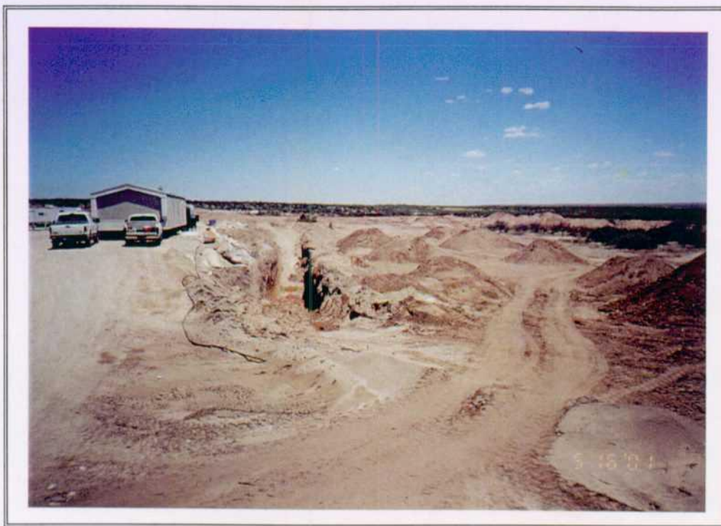
15. Trench #2 - soil excavation and remediation.
