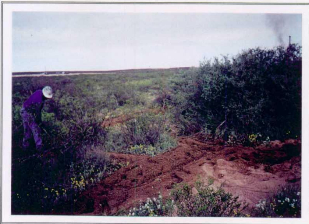
24. Dry Wash - soil remediation, tilling in fertilizer and peat moss.
