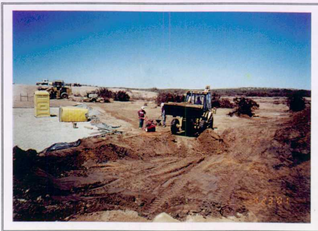
5. Trench #1 - soil excavation and remediation.
