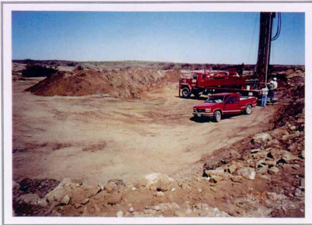
11. Trench #1 - installation of boreholes (BH-5 and BH-6).
