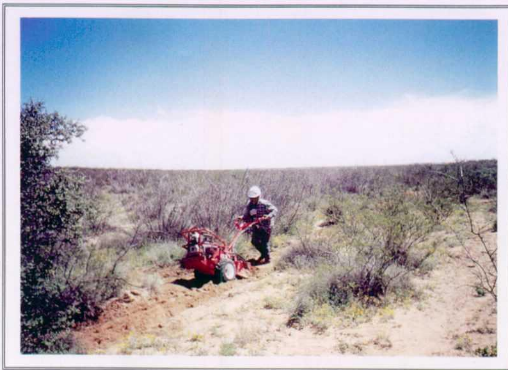
23. Dry Wash - soil remediation, tilling in fertilizer and peat moss.
