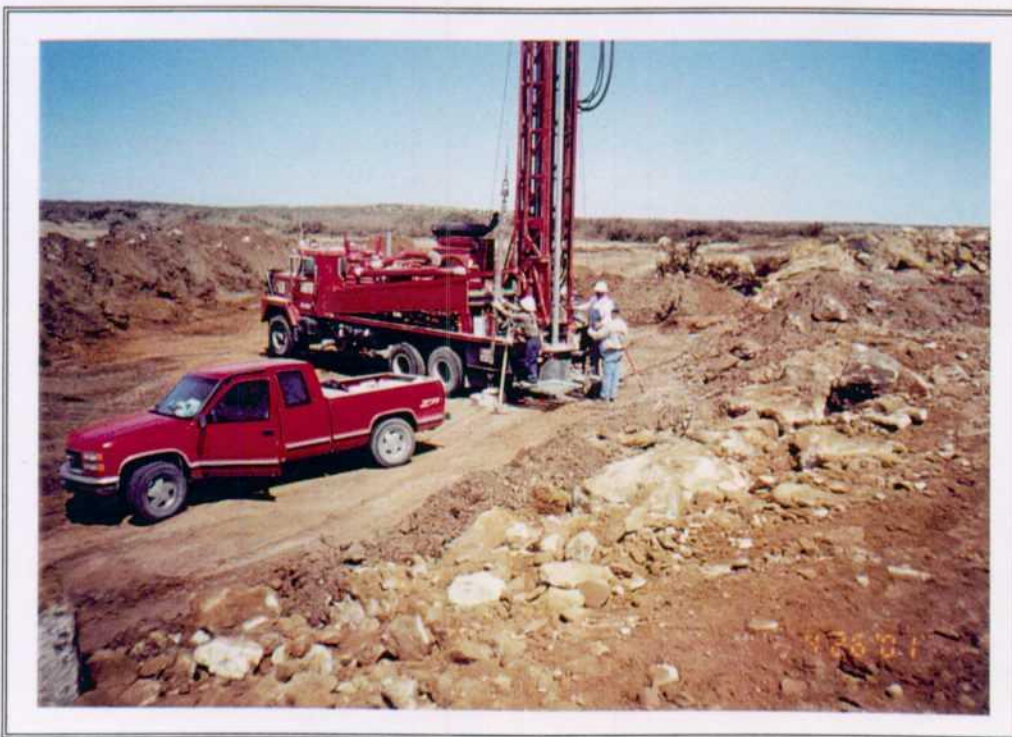
10. Trench #1 - installation of boreholes (BH-5 and BH-6).
